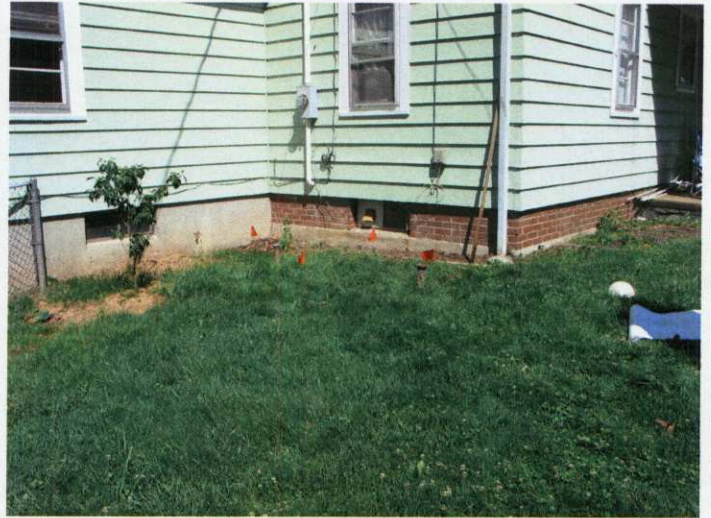
Photograph 2: A closer view, note fill port and vent pipe. Flags outline tank boundaries.
