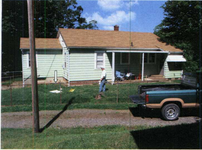
Photograph 1: Looking west at the subject property.
