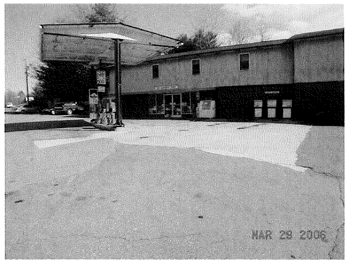
Photograph 2: Area of gasoline, diesel, and kerosene USTs adjacent to subject building and pump island.
