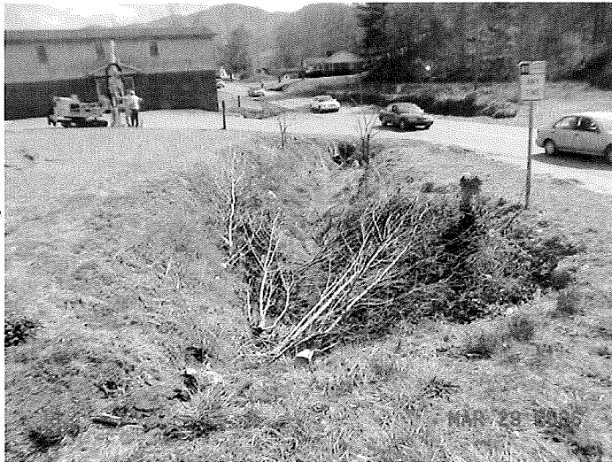
Photograph 3: Drainage culvert on western portion of subject site.
