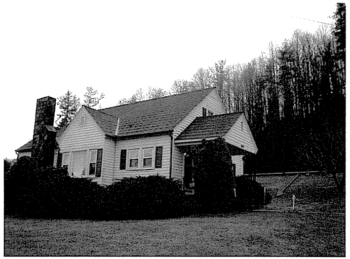
Photograph 2: A closer view. Heating oil UST is located adjacent to far side of porch (See photo).
