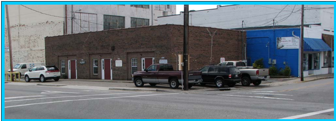
The photograph shows the 601 East Elizabeth Street site (A. Josh Tunnell property - Parcel 17) located at the intersection of East Elizabeth Street and North Poindexter Street in Elizabeth City, North Carolina. The photograph is viewed in a southeasterly direction.
