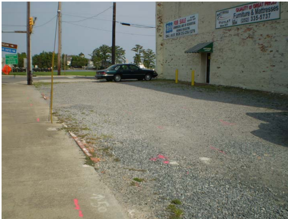
Photograph 2 – View of Value Mart, Inc. property, look east along the former storefront.
