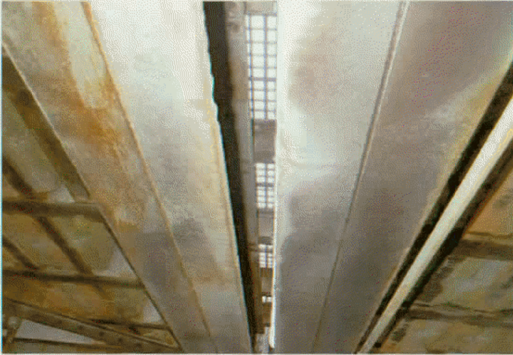
CENTER JOINT BETWEEN EAST AND WEST LIFT
