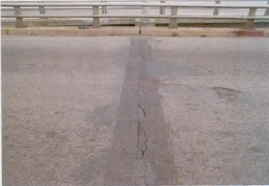
EXPANSION JOINT AT BT#1
