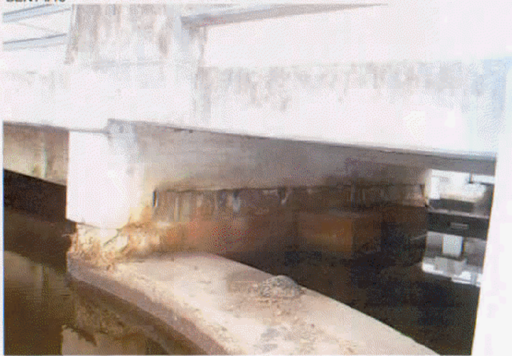
BENT #11 EAST FACE
