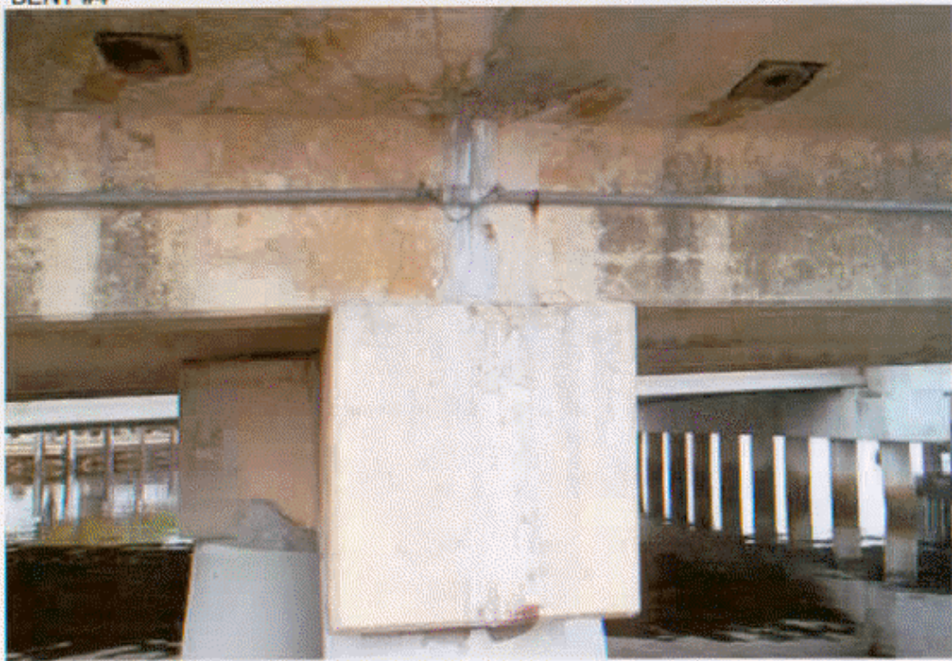
RIGHT END OF BENT #4
