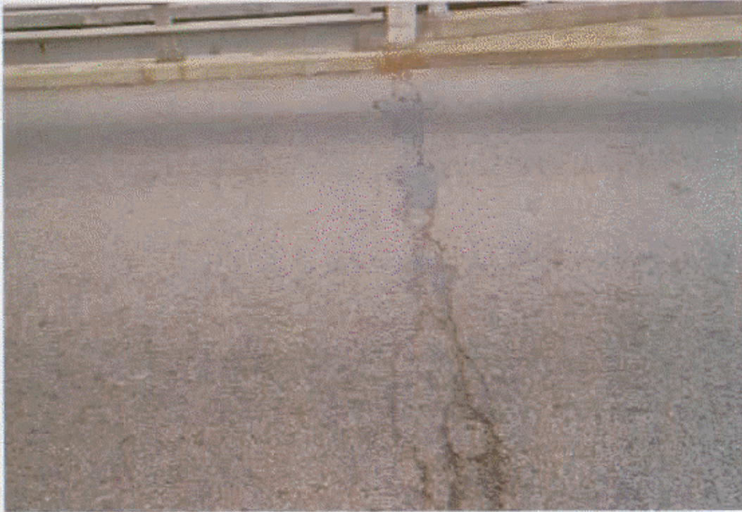
EXPANSION JOINT #4 AT REST PIER#1
