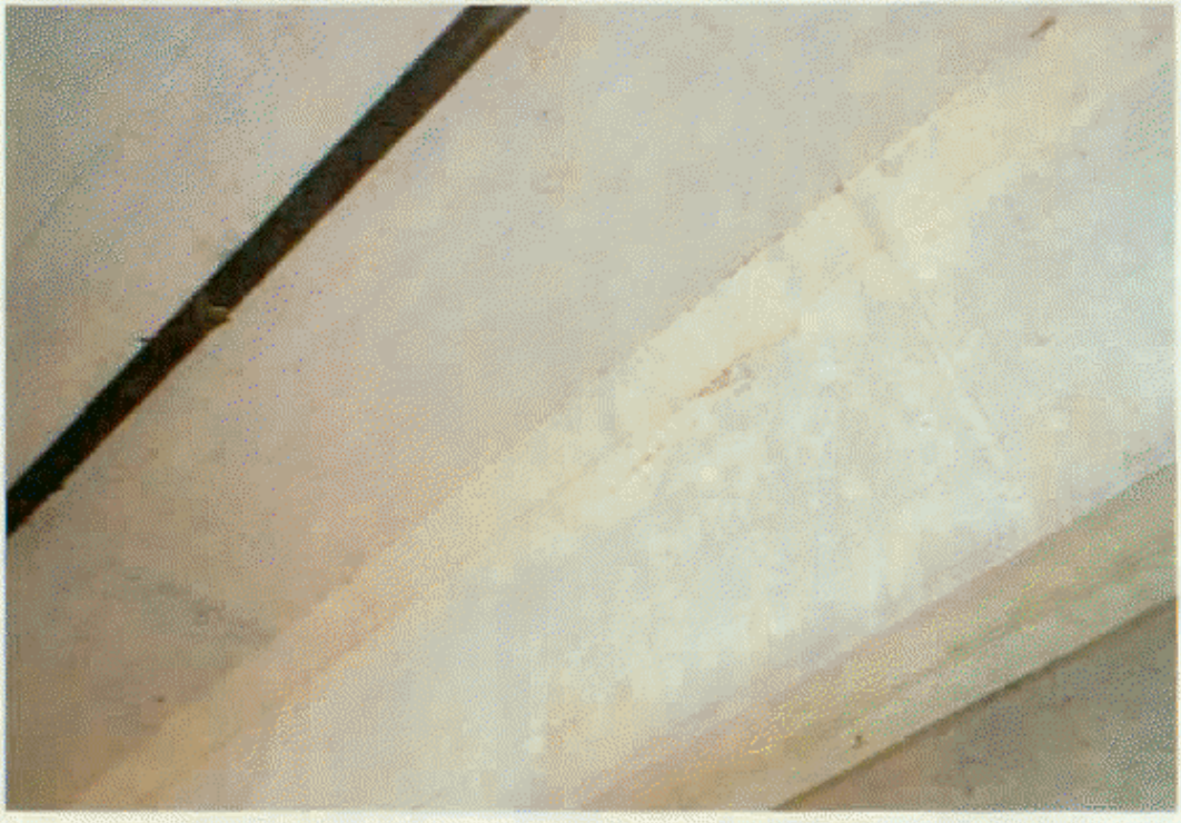
BOTTOM OF DECK
