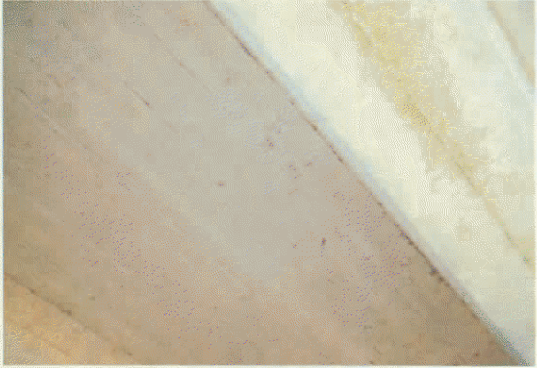
BOTTOM OF DECK
