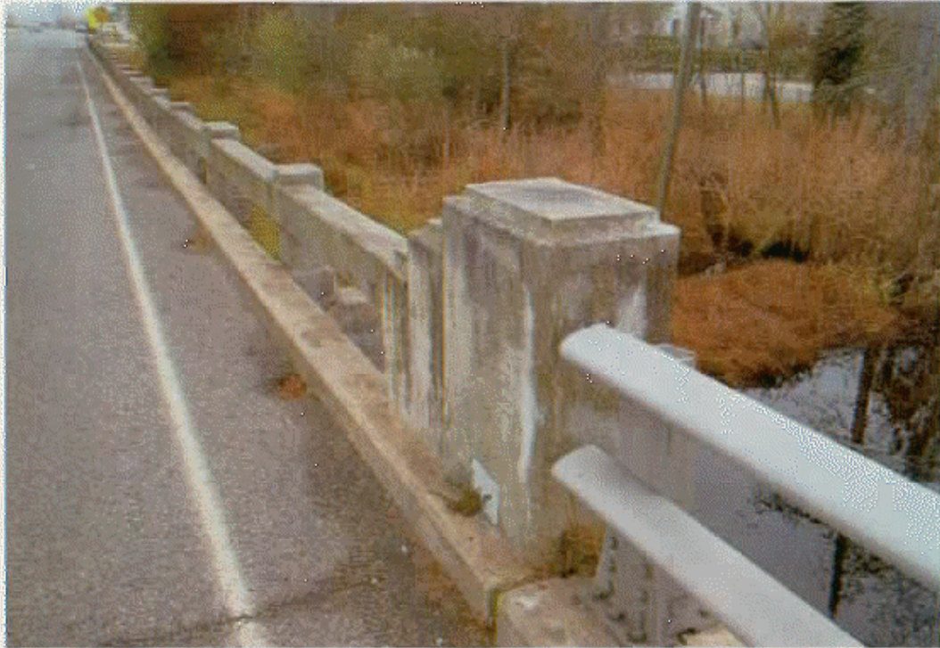
STEEL RAIL STOPS AND RC RAIL STARTS AT BENT#11
