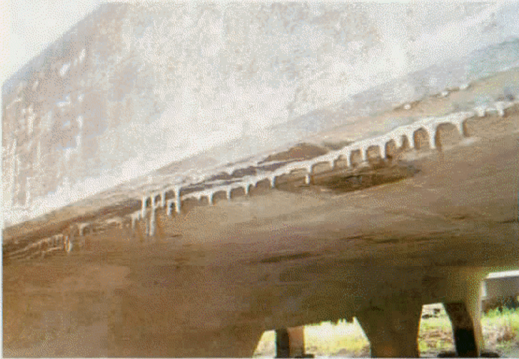
BOTTOM OF DECK (EFFLO)
