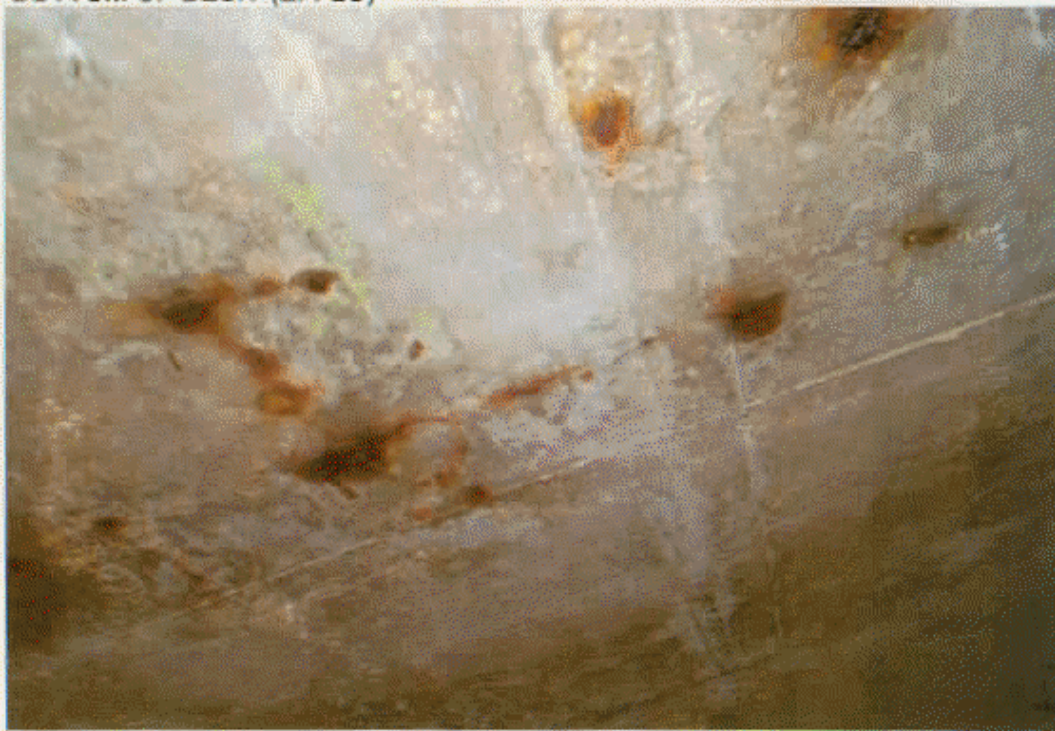
BOTTOM OF DECK
