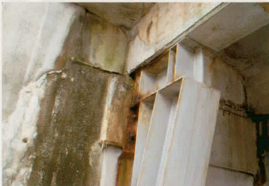
LEFT SIDE OF SUPPORT BEAM AT REST PIER #1 FOR GIRDER #1
