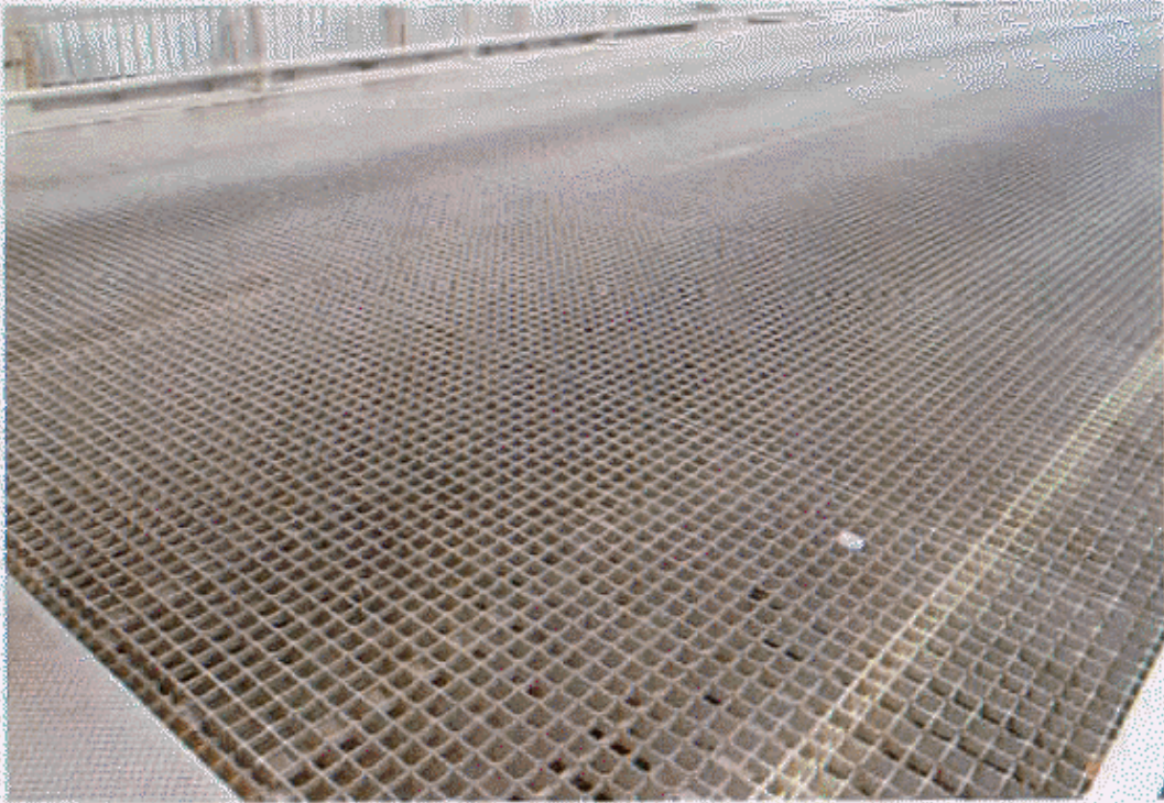
TOP OF STEEL GRID WEST LIFT
