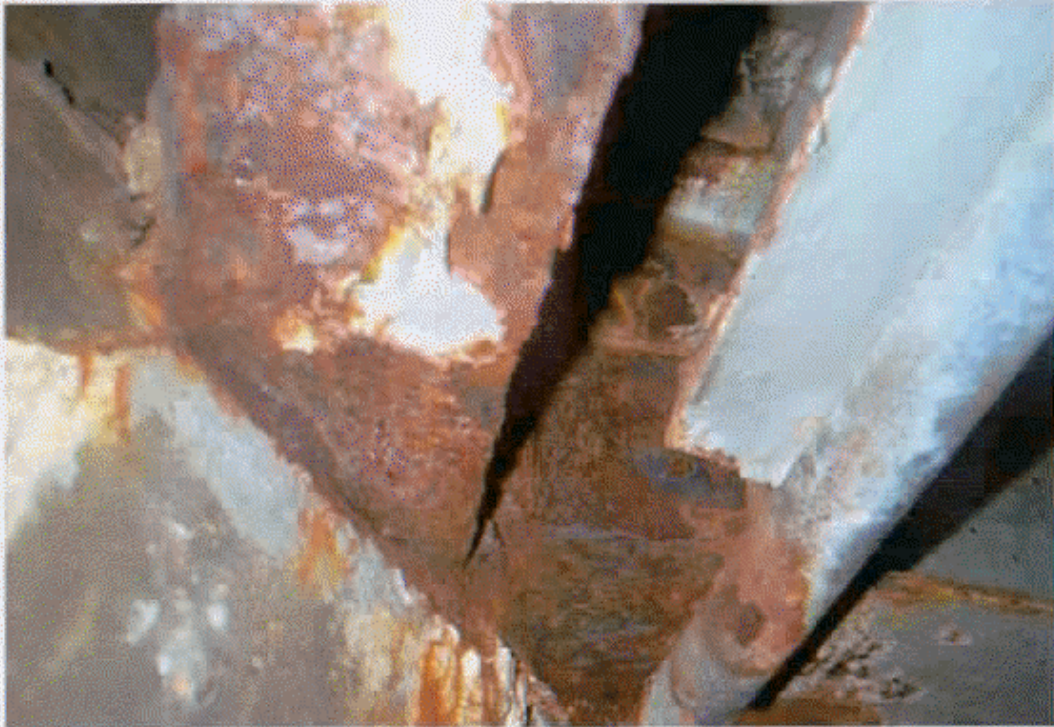
CENTER OF FLOOR BEAM AT BEAM #4 WEST END
