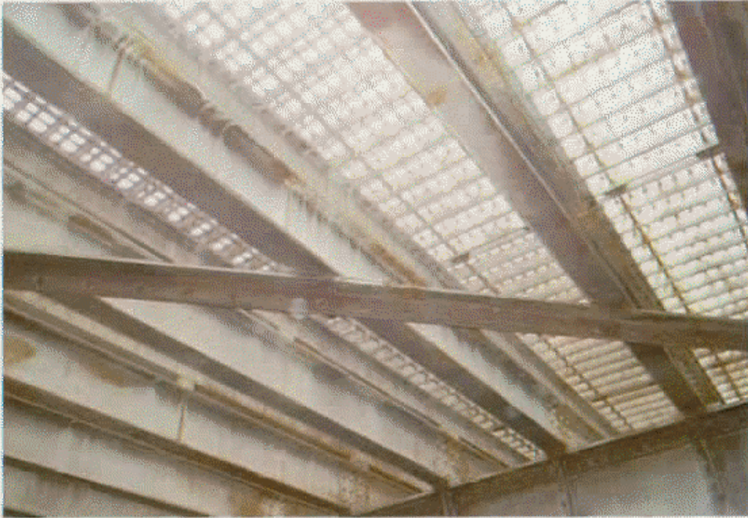
BOTTOM OF STEEL GRID
