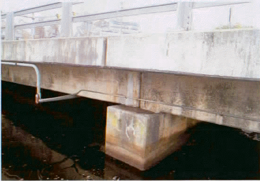
RIGHT END OF BENT #1
