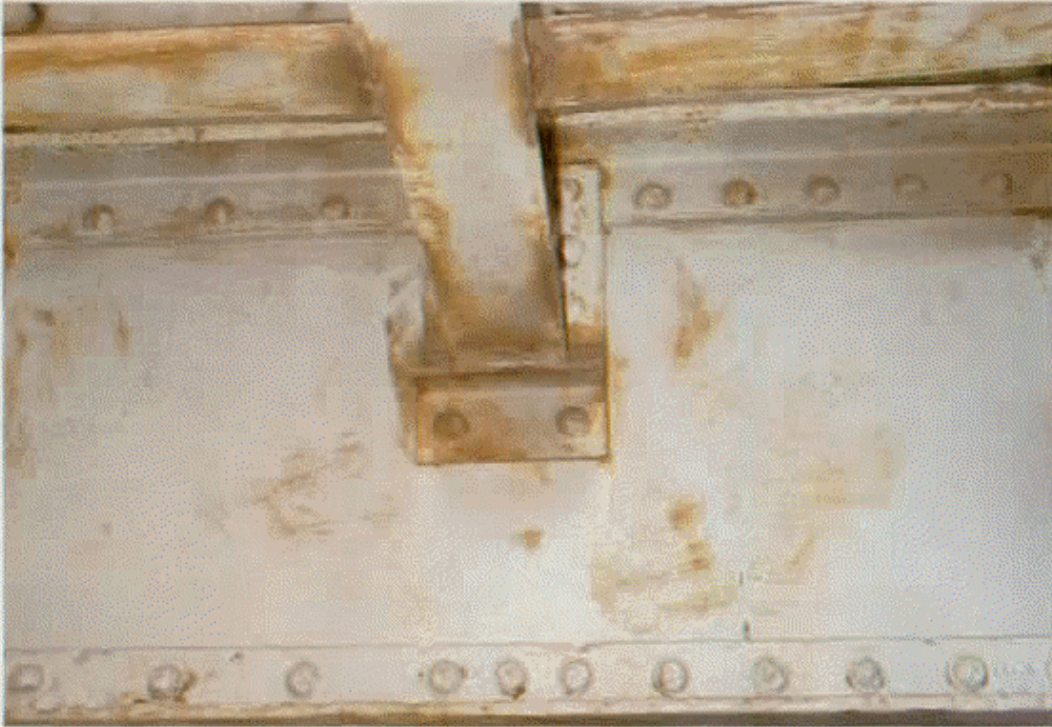
STRINGER ATTACHED TO FLOORBEAM
