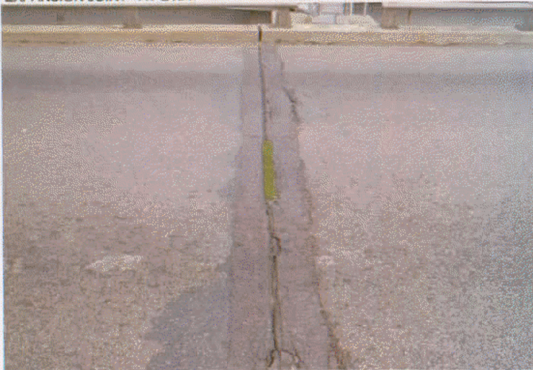
EXPANSION JOINT #3 AT BT#5
