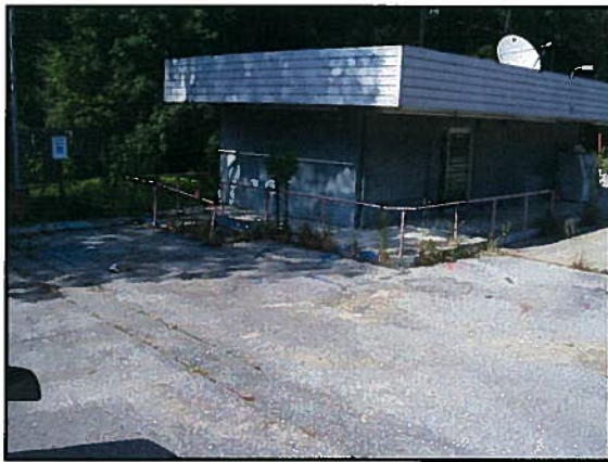
Looking North from UST Basin at former convenience store
