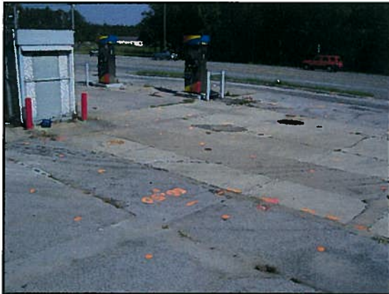
Looking East towards southern dispenser island and across UST basin
