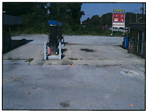
Looking Northeast at northern dispenser island
