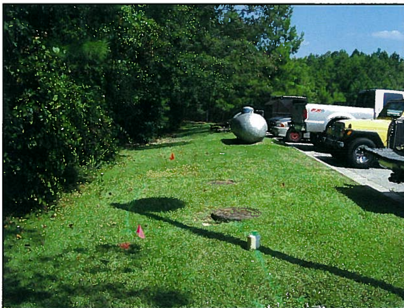
Looking Southwest – Pink flag at DPT-01 – Sewer manholes (2) atop oil-water separator
