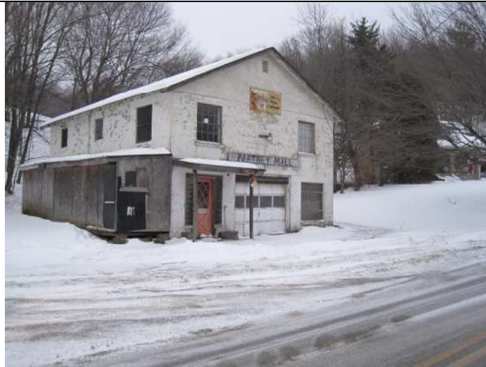
Parcel #34: Matney Mall. View to the south.
