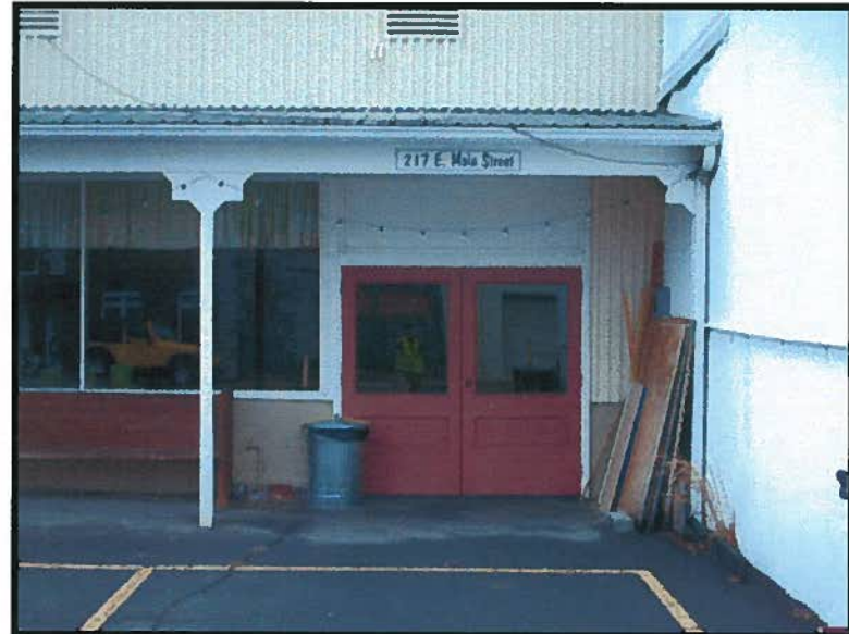
6 View of commercial business on Main Street (rear) portion of Parcel 1 (Vestal Property).
