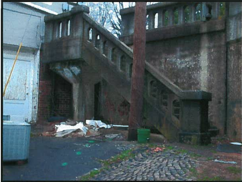
9 View of bridge access on eastern portion of Parcel 2 (Vestal Property).
