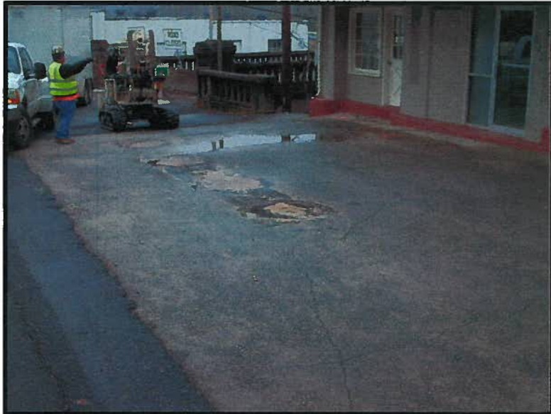
1 Geoprobe operations in front of Parcel 2, Vestal Property.
