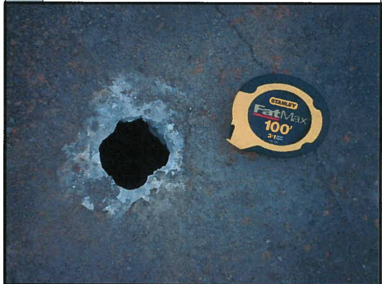
4 View of penetration of suspended slab on Parcel 2, Vestal Property.
