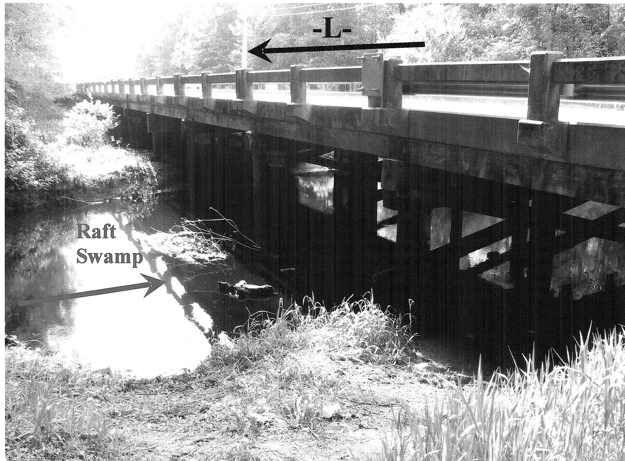
Bridge No. 211 on -L- (SR 1527) Over Raft Swamp
