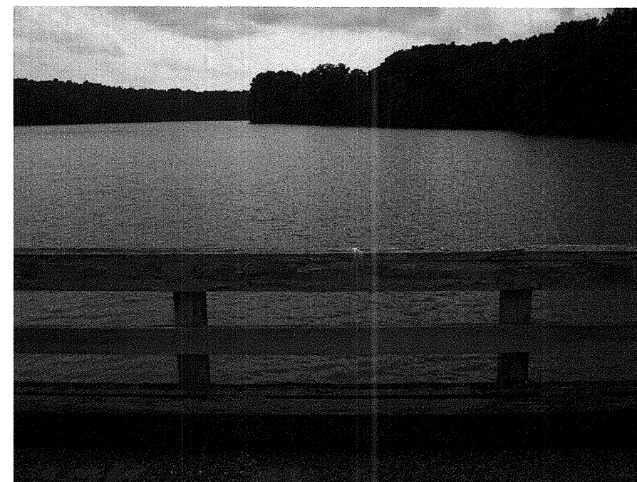
Photograph No. 4: This photograph was taken from the centerline of the -L- alignment, looking west, across proposed Interior Bent No. 1.
