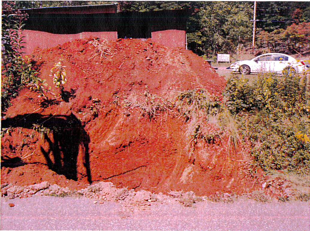
Photograph 3: Soil excavation and stockpile
