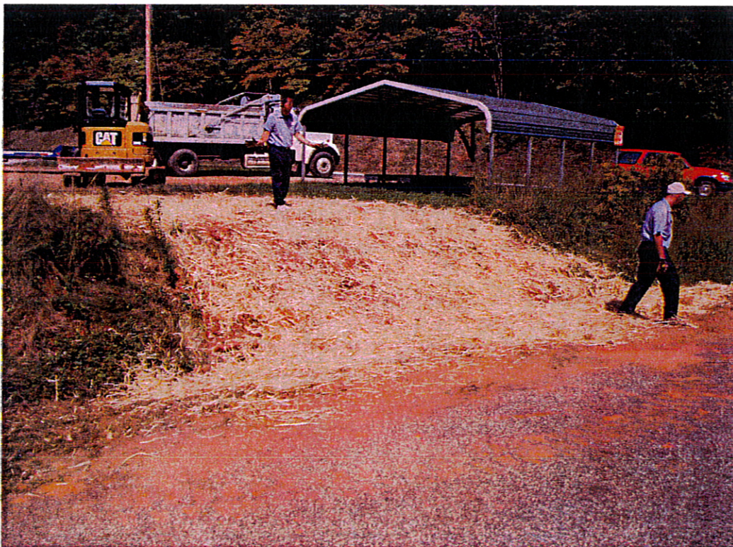
Photograph 4: View of area after exploratory excavation
