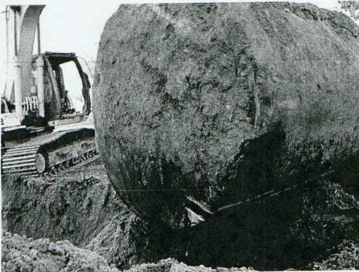
02060548 Former Esso/Exxon (Register Property) Tank #1-No holes, good condition
