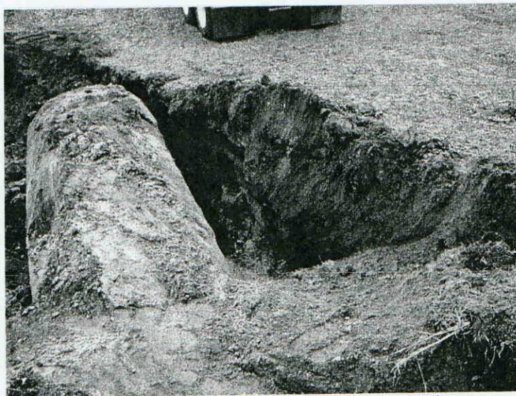
02060548 Former Esso/Exxon (Register Property) Tilted USTs to remove remaining liquid
