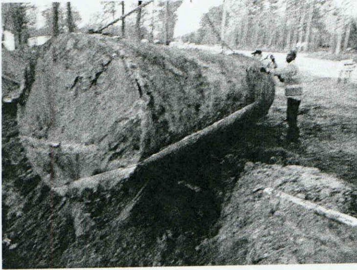
02060548 Former Esso/Exxon (Register Property) Tank #1
