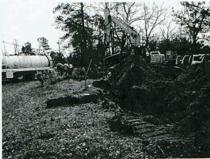
02060548 Former Esso/Exxon (Register Property) Begin removing liquid from USTs
