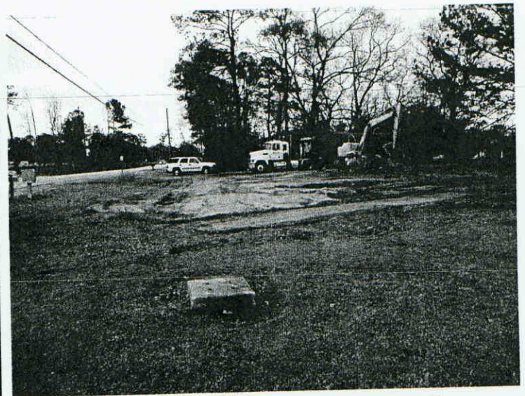
02060548 Former Esso/Exxon (Register Property) All tank beds backfilled
