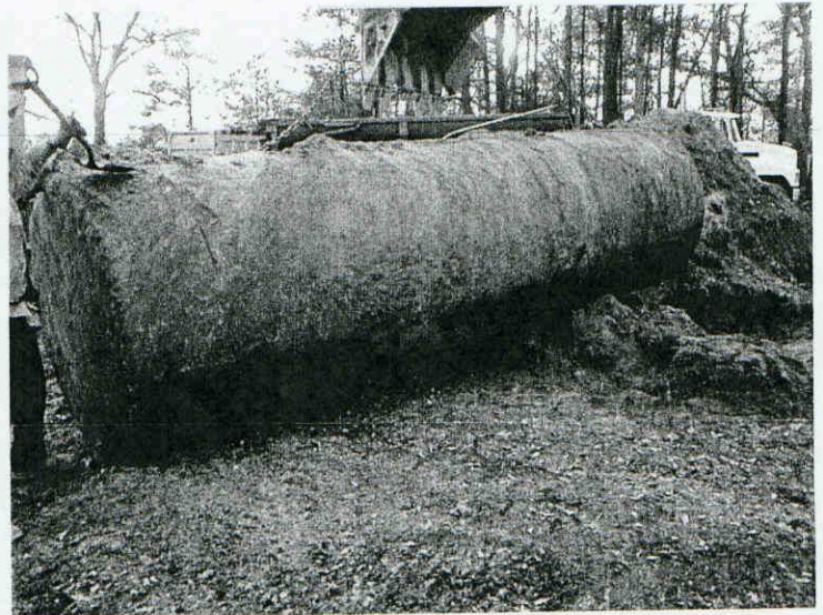
02060548 Former Esso/Exxon (Register Property) Tank #2- 64"X18'
