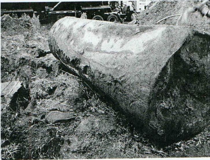
02060548 Former Esso/Exxon (Register Property) Tank #4-No holes, good condition
