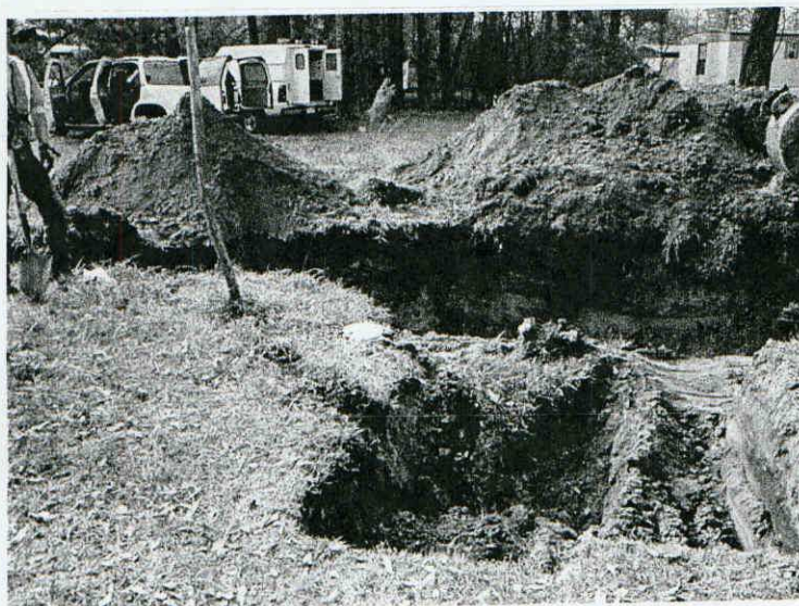
02060548 Former Esso/Exxon (Register Property) Unearthing Tank #1 and Tank #2
