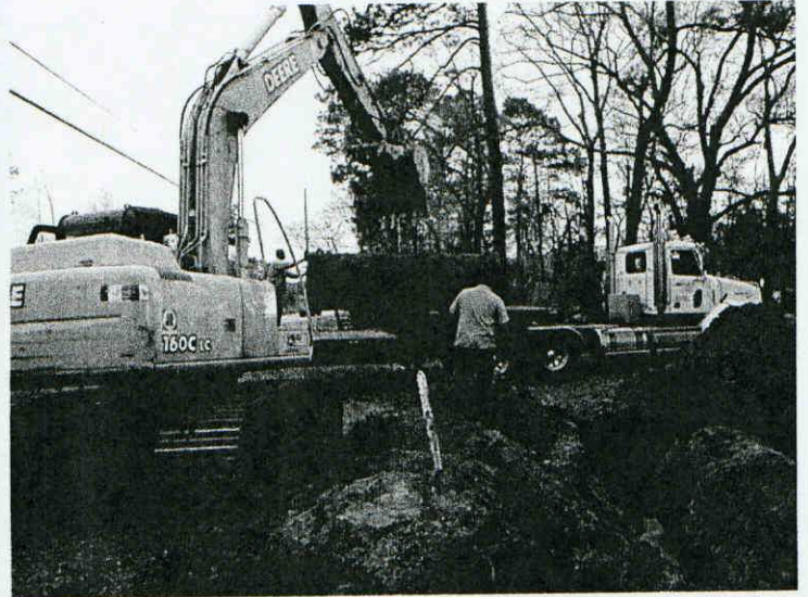
02060548 Former Esso/Exxon (Register Property) Loading Tank #4- Measured 46"X12'
