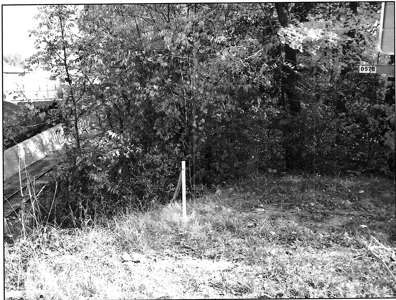
BENT 4, LOOKING LEFT TO RIGHT FROM WILSON LEE BLVD.
