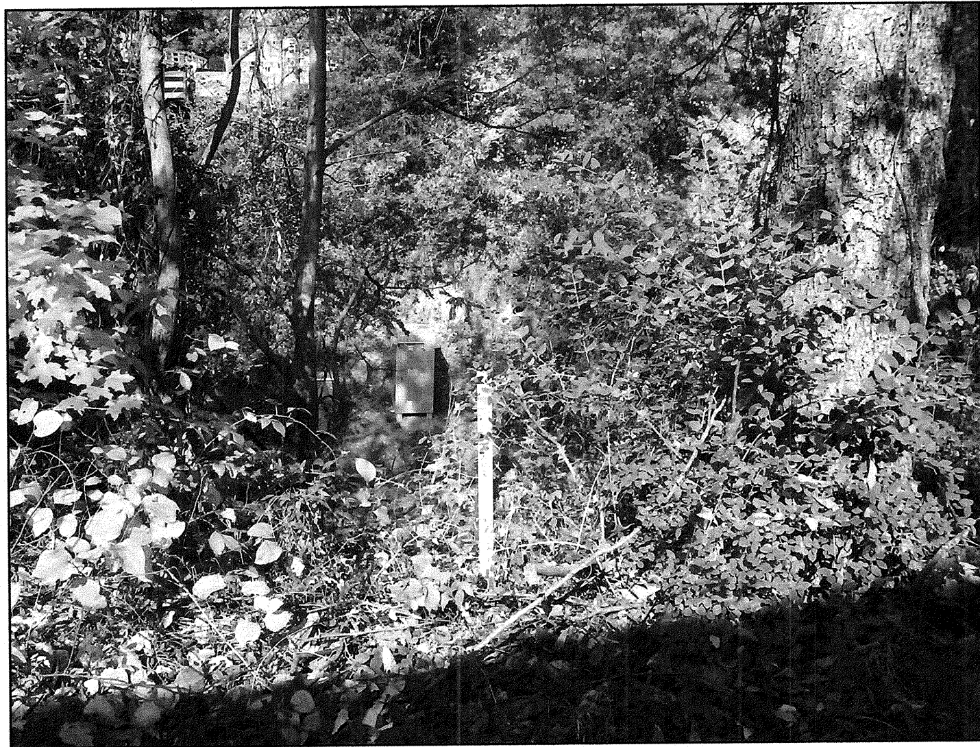
LOOKING TOWARDS BENT 3 FROM BENT 2 AREA. NOTE EXPOSED SOIL SURFACES ON SLOPE.
