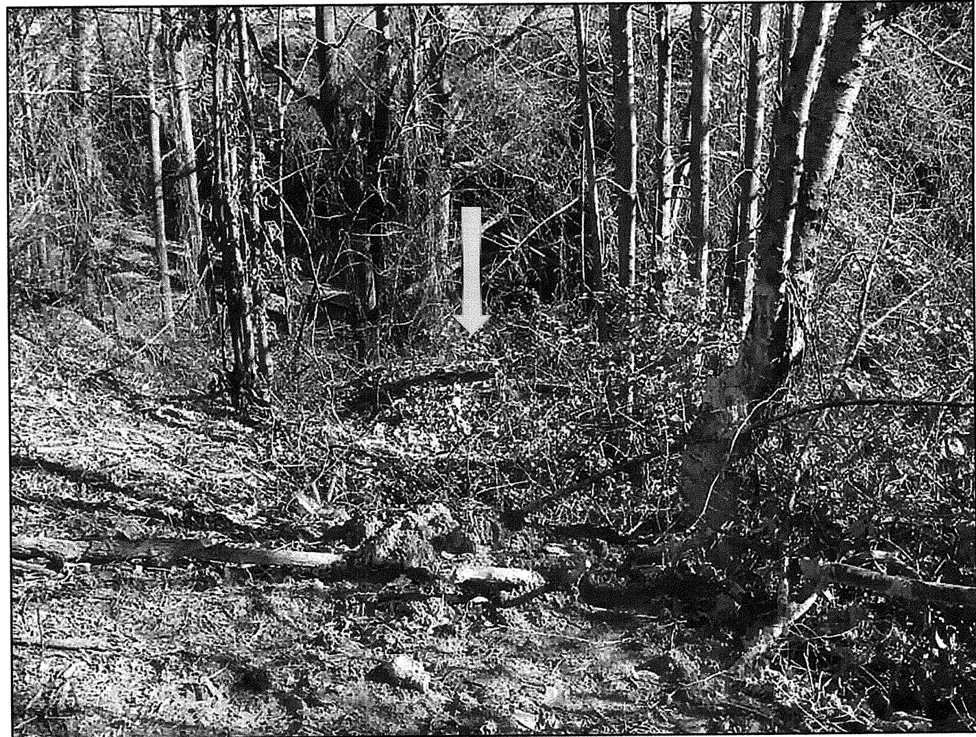
POTENTIAL SLUMP BLOCK, LOOKING SOUTHEAST FROM B3-B. GRAY ARROW POINTS TO SLUMP BLOCK SURFACE.
