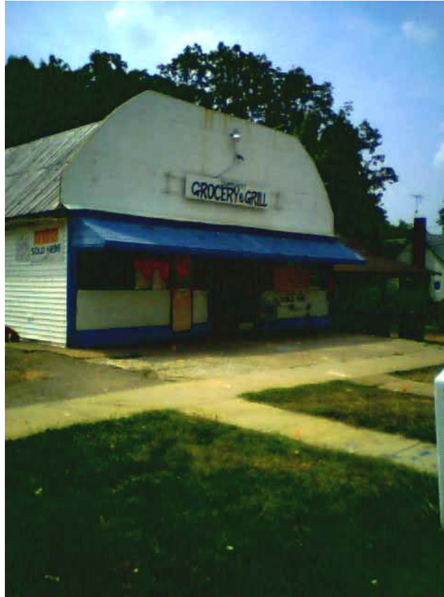
Photograph 1 – View toward the west of the James Hunter Property.
