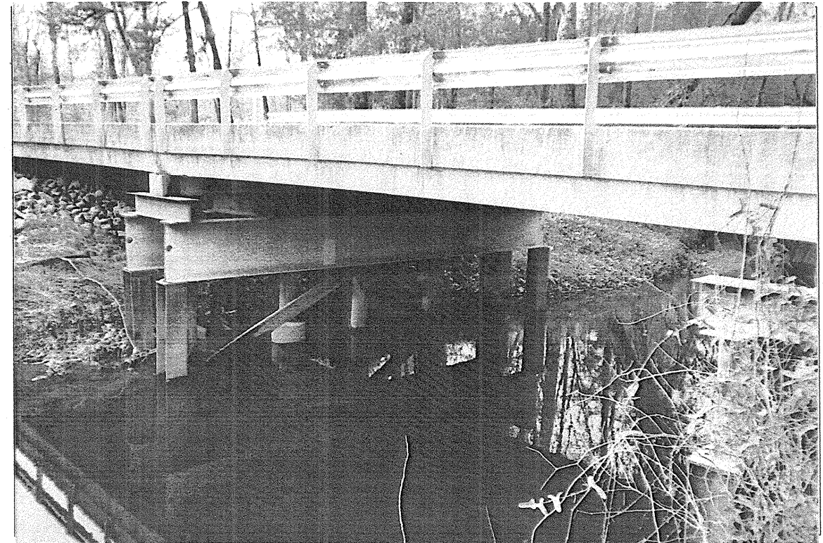
Photograph No. 3: Looking northwest from end bent 2.
