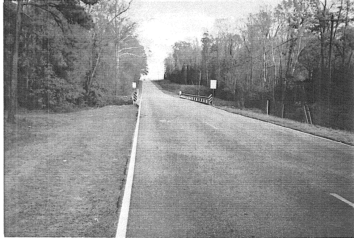
Photograph No. 1: Looking east along SR 1091.
