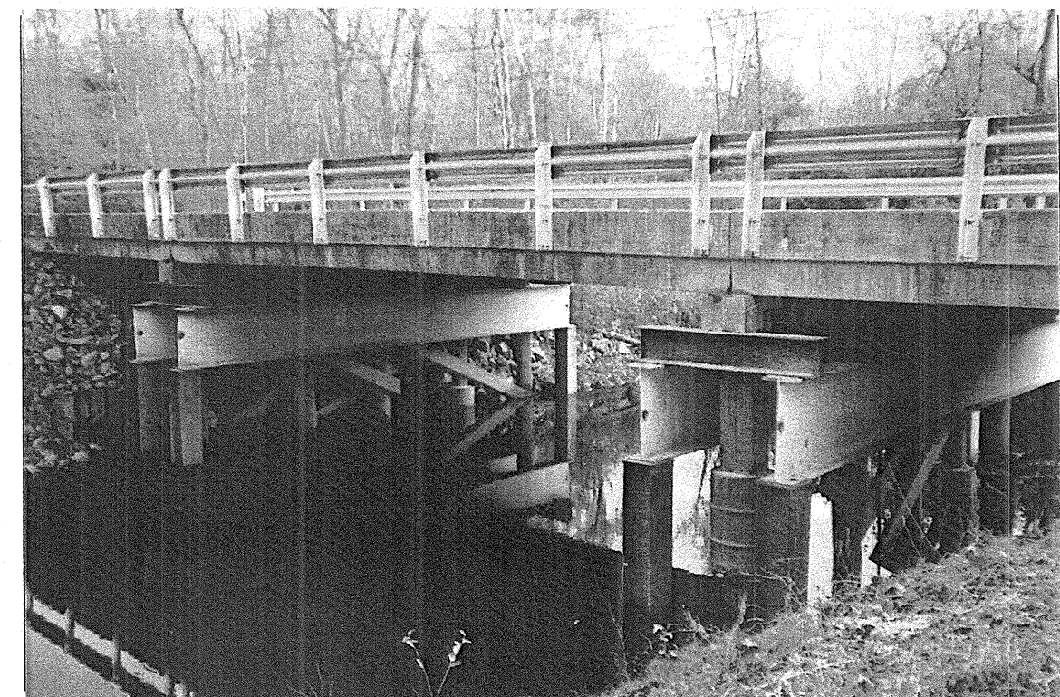
Photograph No. 4: Looking southeast from end bent 1.
