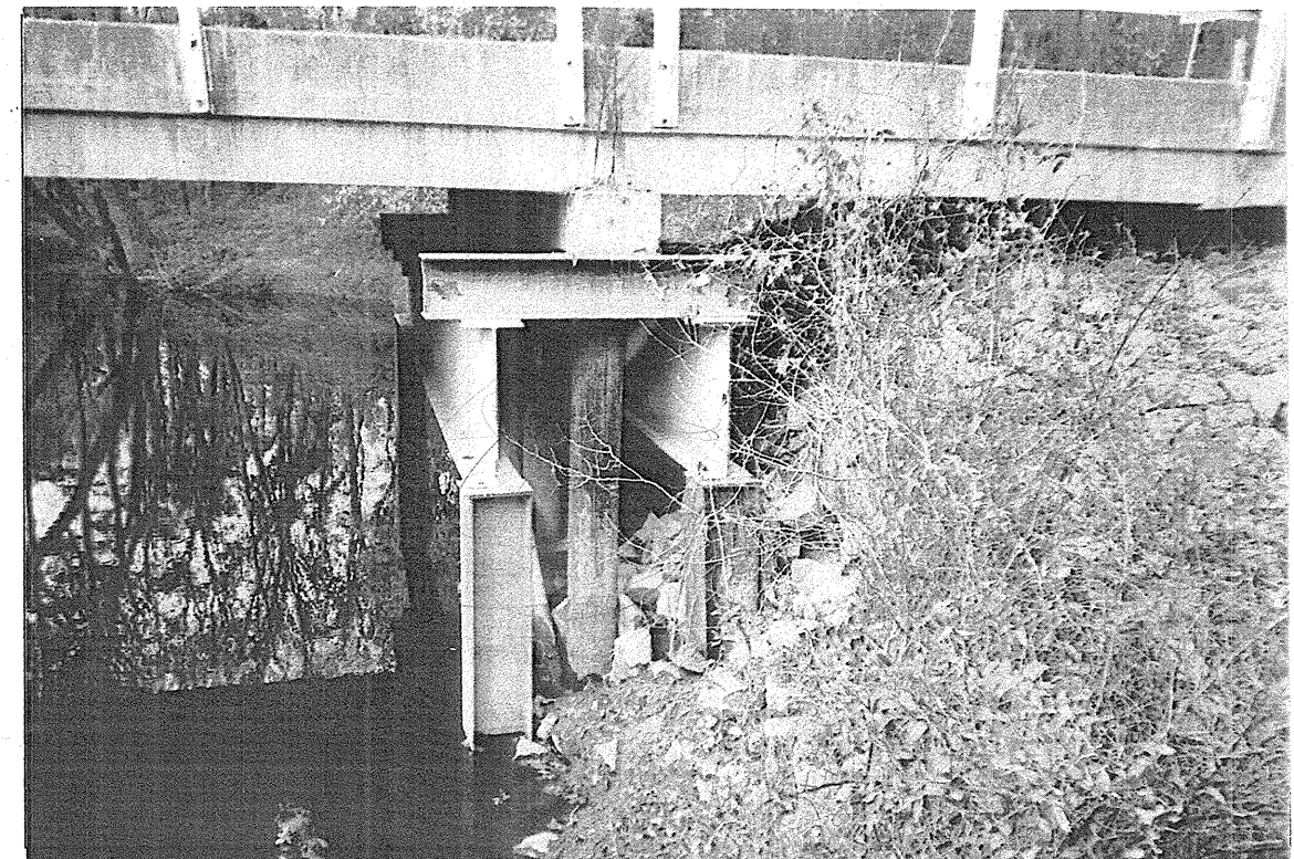
Photograph No. 7: Looking north along bent 2.
