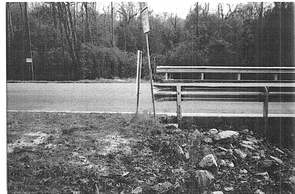
Photograph No. 8: Looking south along end bent 2.
