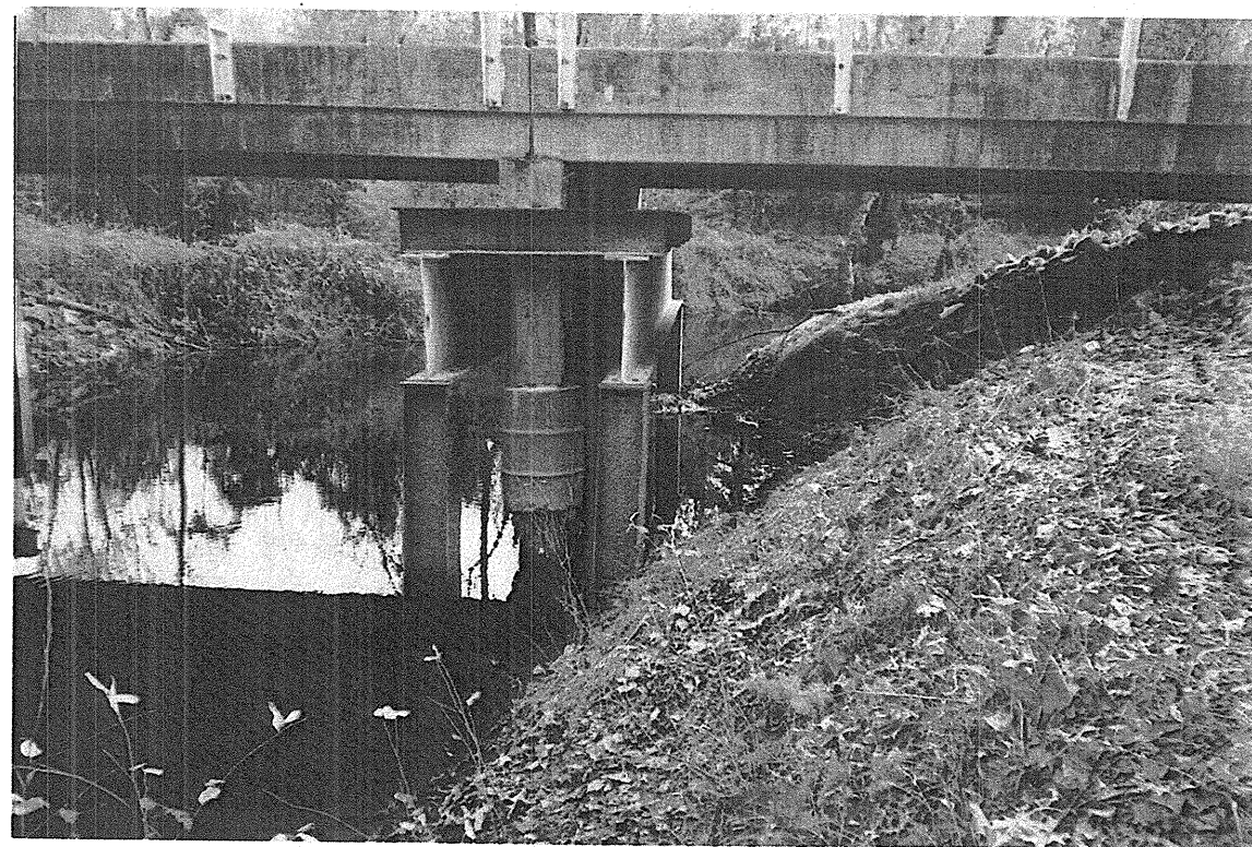
Photograph No. 6: Looking south along bent 1.
