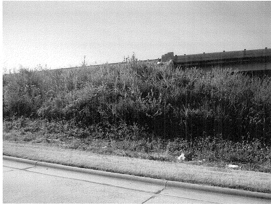
Photograph No. 5: This photograph was taken at the toe of the existing embankment, from the right side of the -L- alignment, looking south, across proposed End Bent No. 1.
