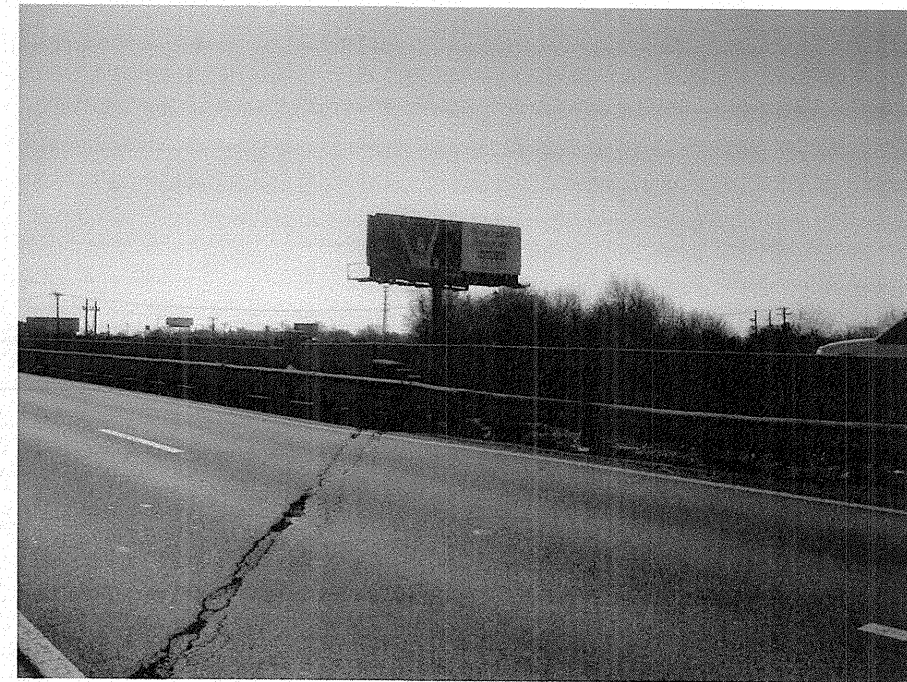
Photograph No. 15: This photograph was taken at the top of the existing embankment, from the right side of the -L- alignment, looking south, across proposed End Bent No. 2.
