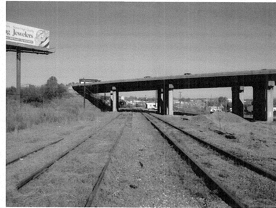
Photograph No. 11: This photograph was taken from the left side of the -L- alignment, along the Norfolk Southern Railroad tracks, looking north.
