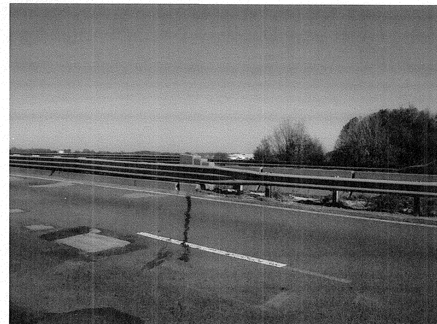
Photograph No. 4: This photograph was taken at the top of the existing embankment, from the left side of the -L- alignment, looking north, across proposed End Bent No. 1.
