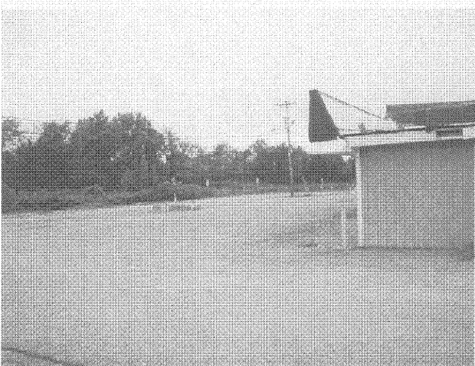
Photograph 5: View of parcel frontage looking northwest.
