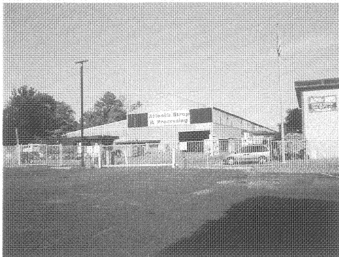
Photograph 1: View of subject property.
