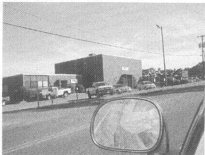
Photograph 1: View of subject property.
