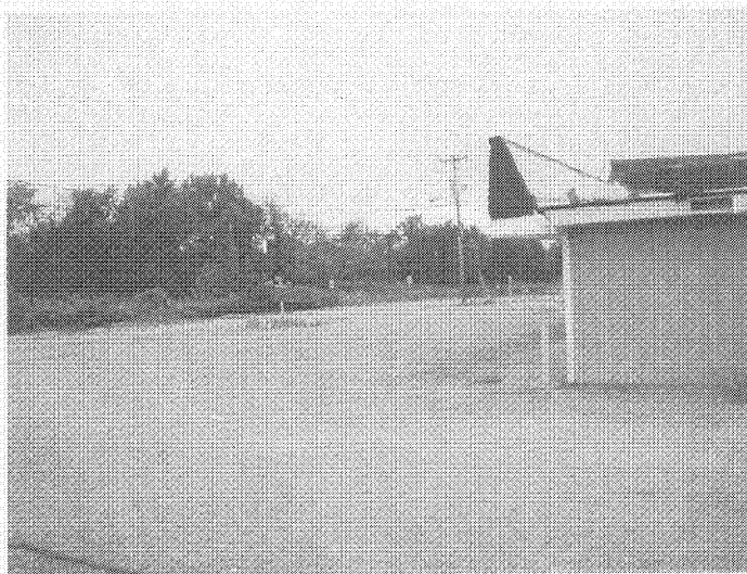
Photograph 5: View of parcel frontage looking northwest.
