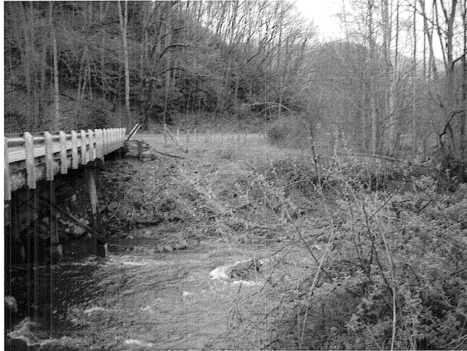
View looking down station along -L- towards proposed End Bent 1
