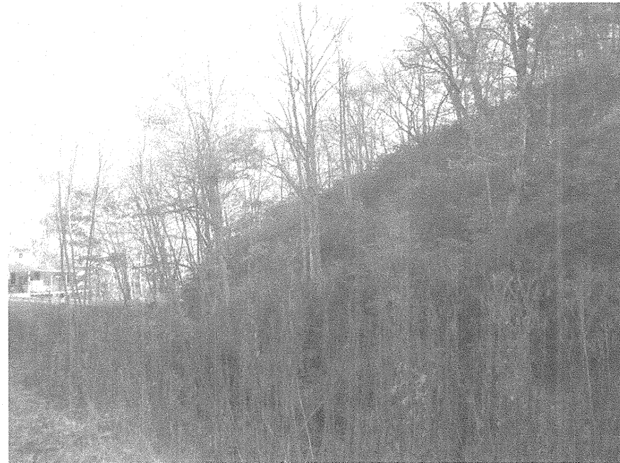
Photograph No. 1: This photograph was taken from the west approach at approximately Station 11+00, looking northeast at the slope to be cut relative to the New River General Store.
