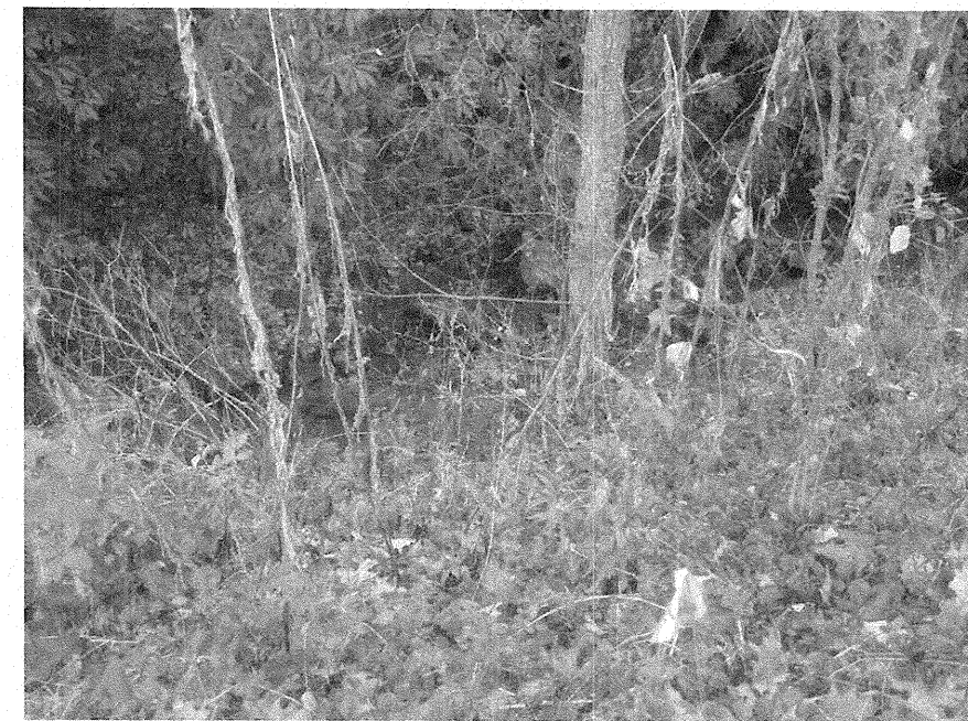
Photograph No. 4: This photograph was taken at approximately Station 13+00, looking southeast (right) at the existing stream bed south of existing 6'X6' concrete box culvert headwall.
