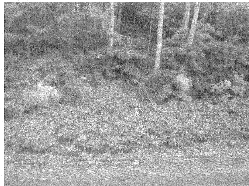
Photograph No. 6: This photograph was taken at approximately Station 14+00, looking south (right) at the existing slope with rock outcrops.
