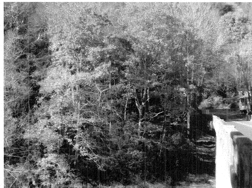
Photograph No. 10: This photograph was taken from the east approach, looking west at the existing slope to be cut relative to the New River General Store.
