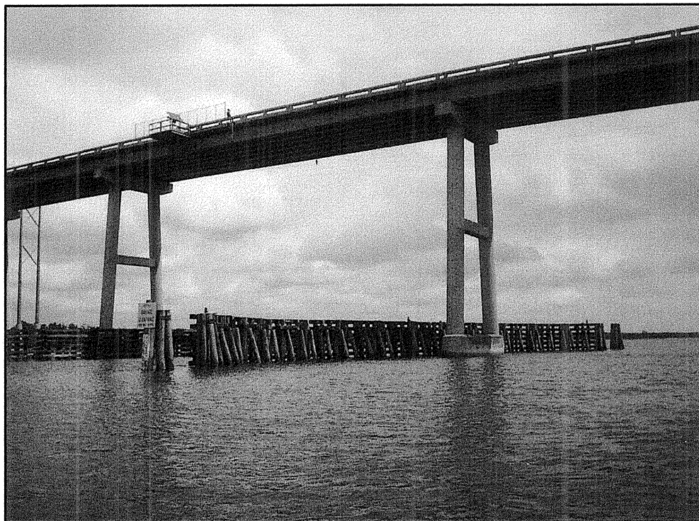
WEST OF BRIDGE #6 FACING ENE SOUTH FENDER IN FOREGROUND
