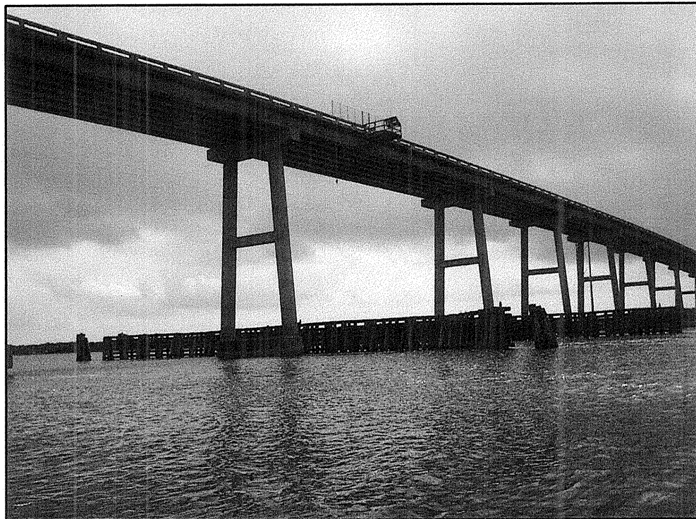
WEST OF BRIDGE #6 FACING SE NORTH FENDER IN FOREGROUND
