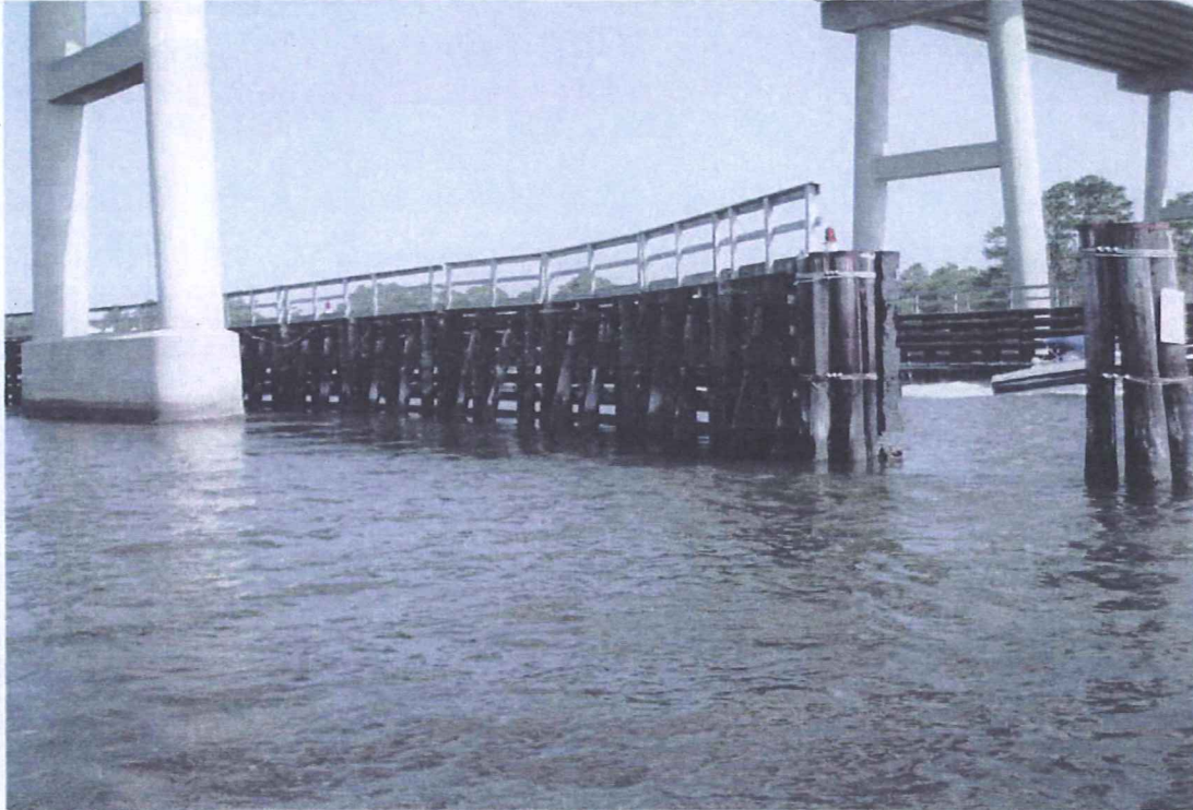
BACKSIDE SOUTH FENDER
