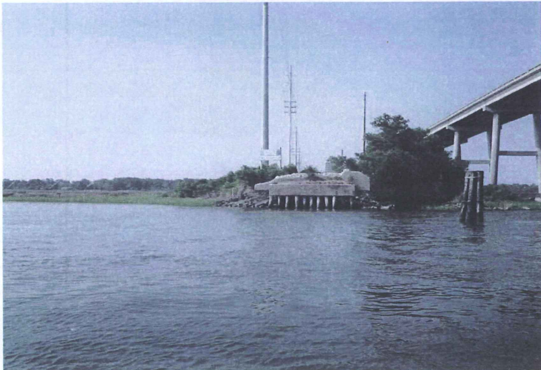
CABLE CROSSING SIGN
