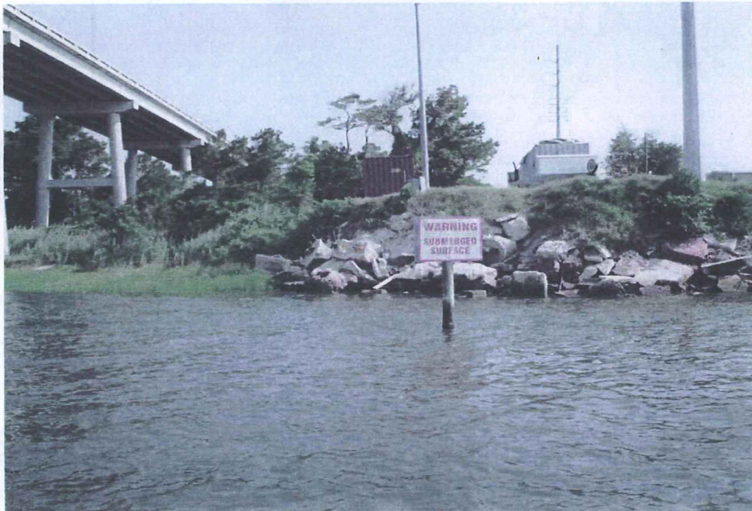
WARNING SIGN NORTHWEST CORNER
