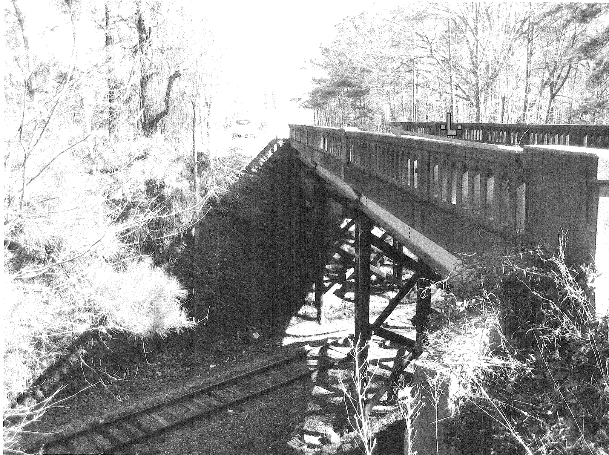
Looking East towards End Bent 2
