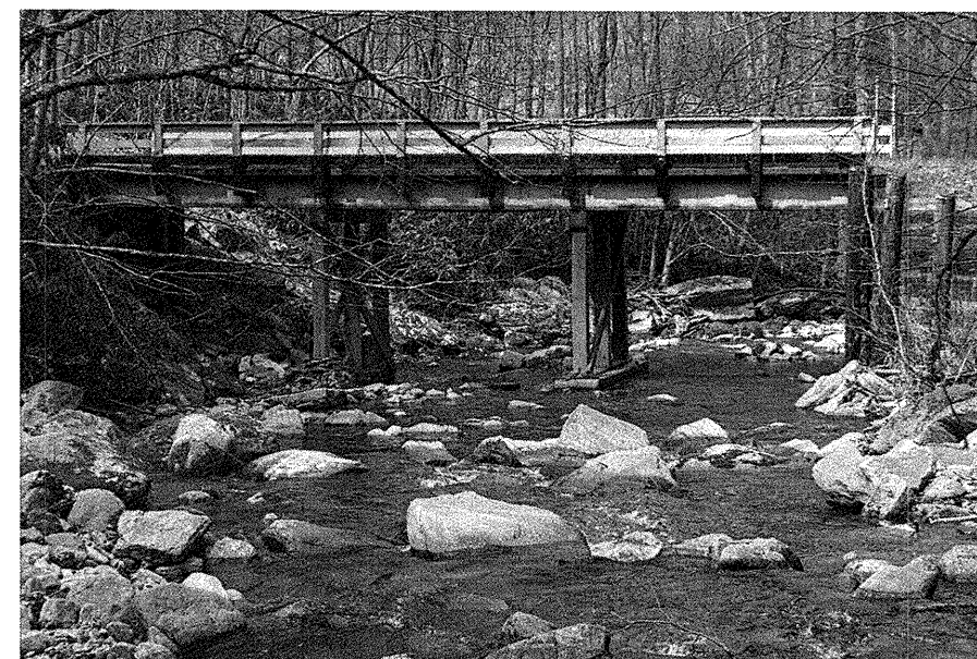
Photograph No. 4 - Proposed Bridge looking west downstream at the Existing Bridge
