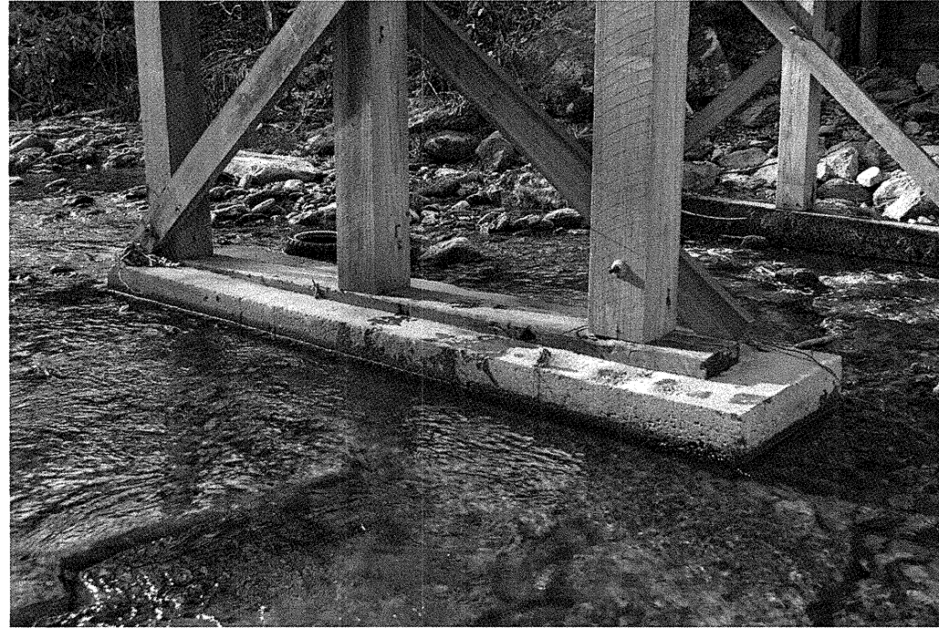
Photograph No. 1 - Bent 3 (north side) foundation & piers
