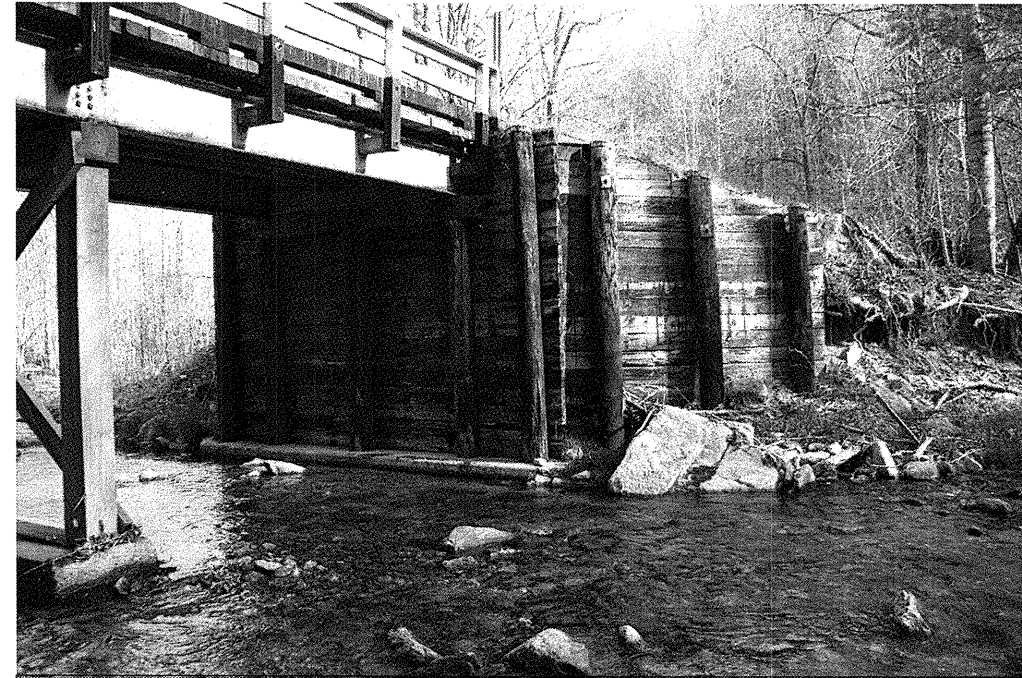
Photograph No. 3 - North (bent 4) abutment upstream wingwall
