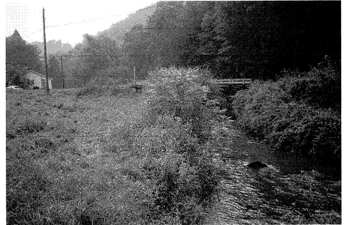
Fig. 1: Looking Upstream at Culvert.
