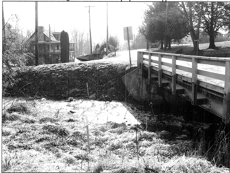
Photo-2: Looking upstation at -L- proposed from approximate EB1-C
