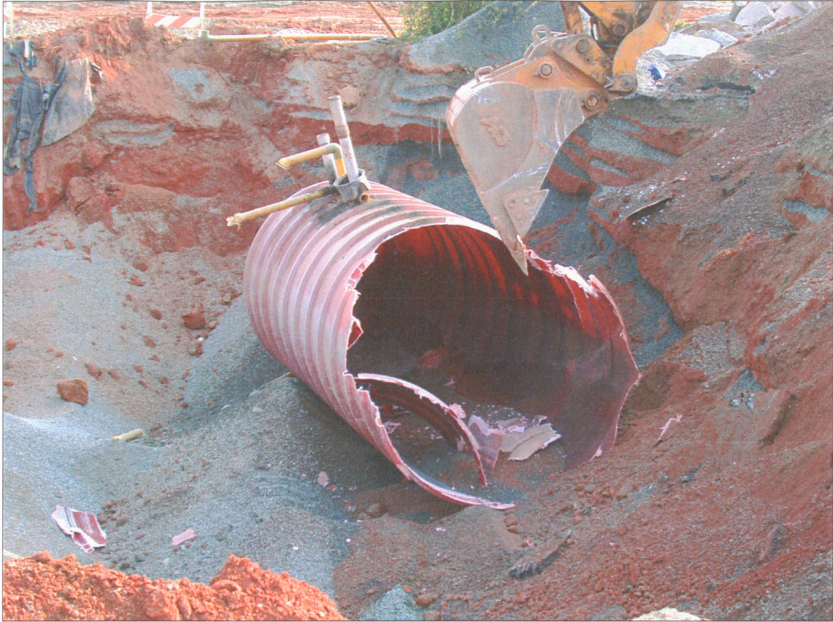
PHOTO 9 - 15,000-GALLON UST DEMOLISHED
