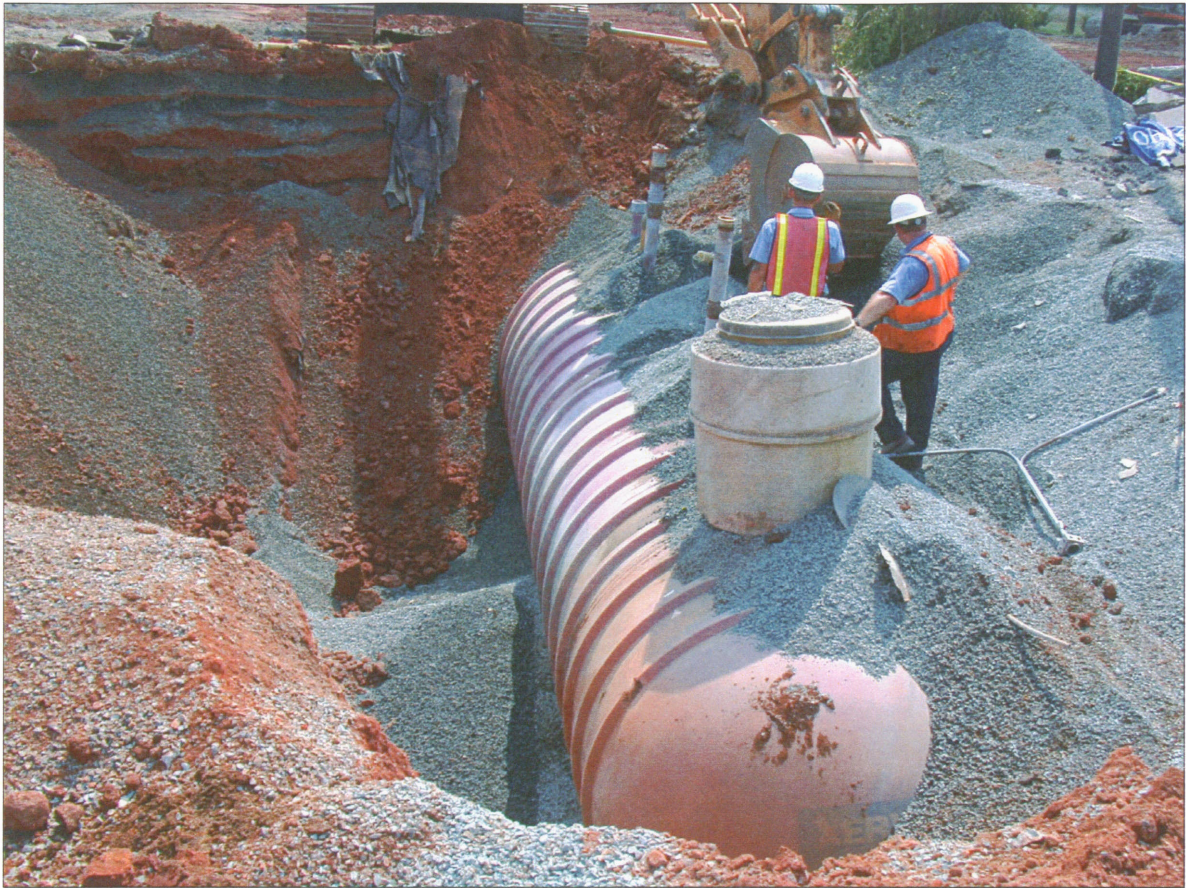
PHOTO 5 - 10,000-GALLON UST UNCOVERED
