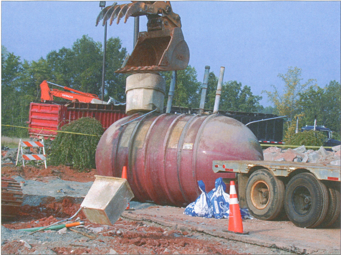
PHOTO 3 - 4,000-GALLON UST OUT OF THE GROUND
