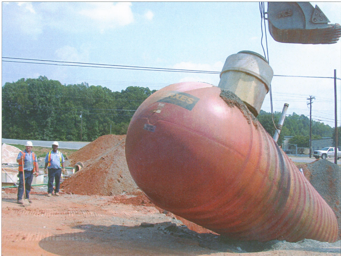
PHOTO 6 - 10,000-GALLON UST OUT OF THE GROUND
