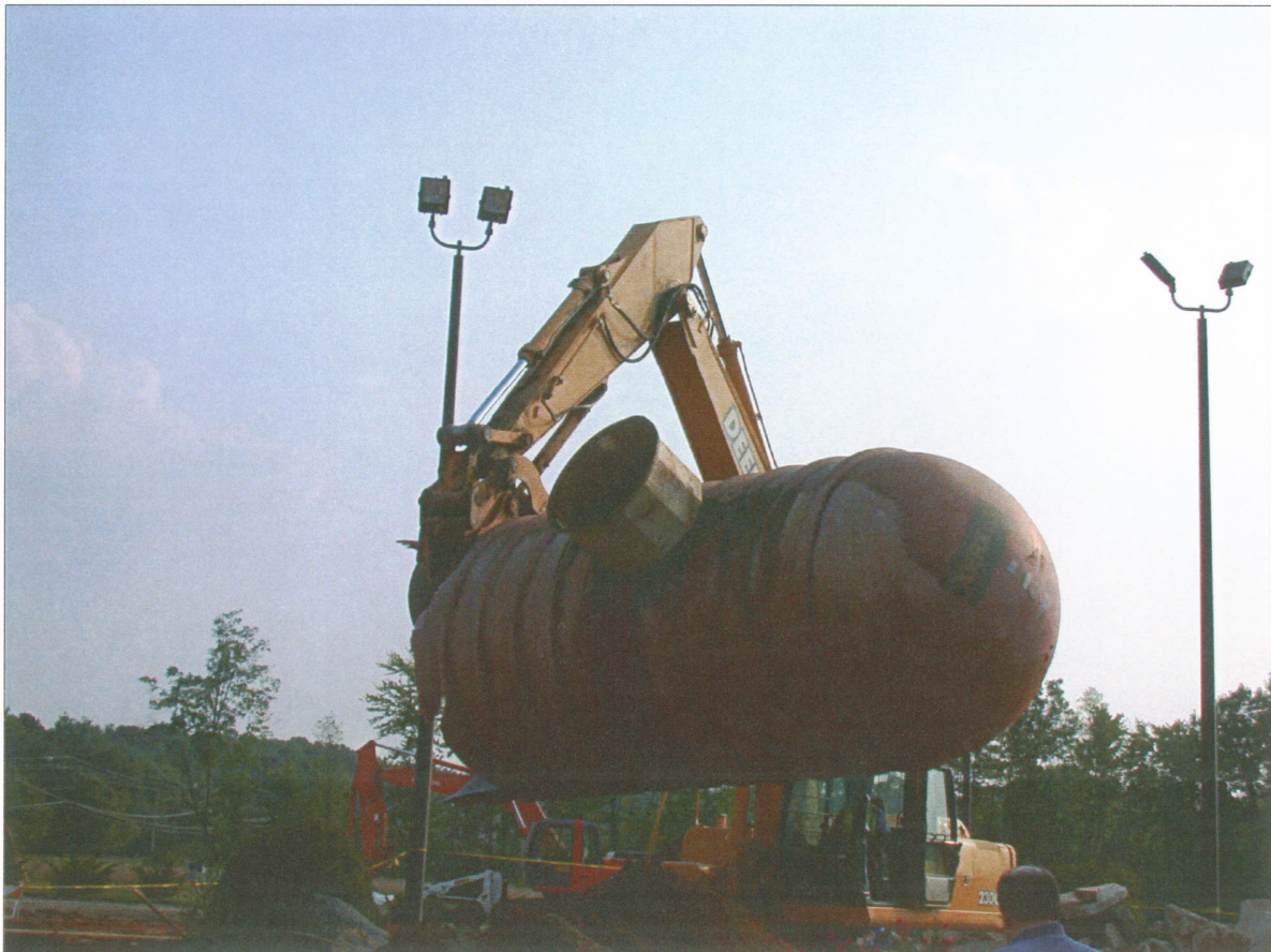
PHOTO 8 - 15,000-GALLON UST PARTIALLY DEMOLISHED
