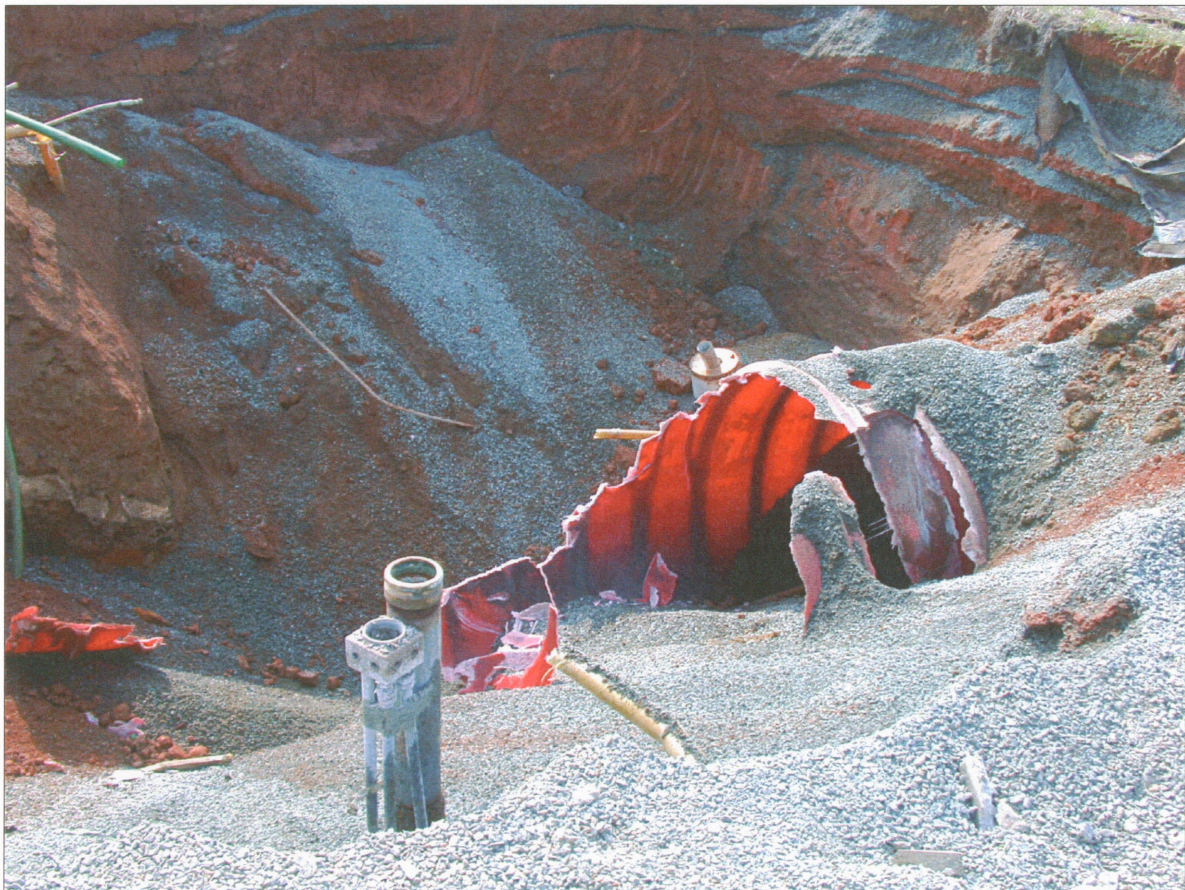
PHOTO 4 - 8,000-GALLON UST DEMOLISHED IN-PLACE
