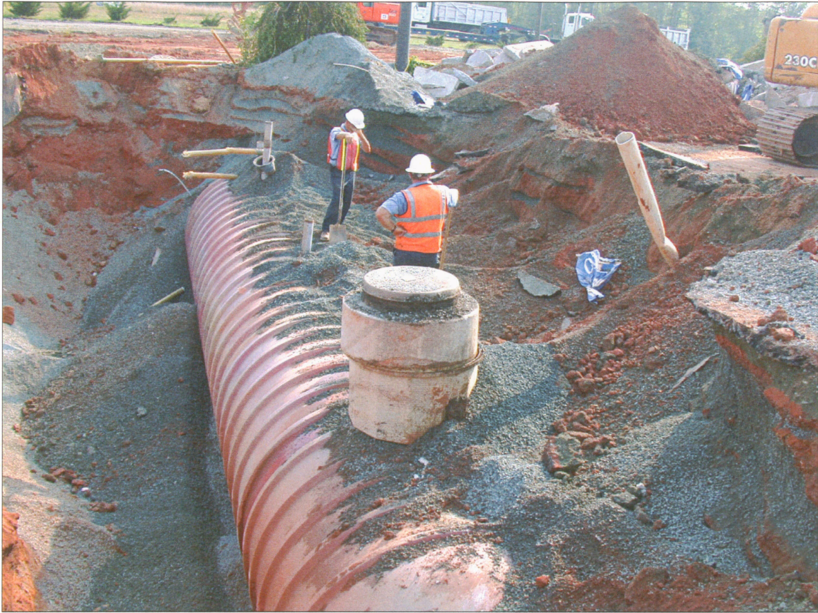
PHOTO 7 - 15,000-GALLON UST UNCOVERED
