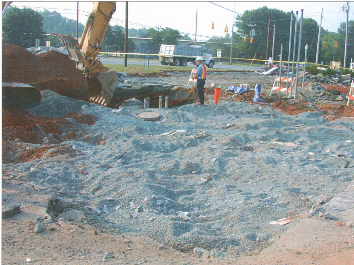
PHOTO 2 - UST AREA PRIOR TO EXCAVATION
