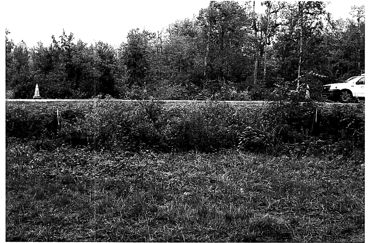
View looking right to left along End Bent 1.
