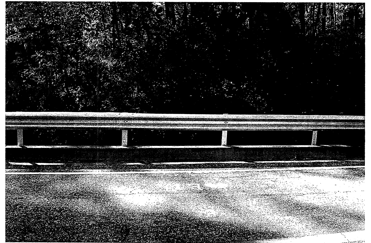
View looking left to right along Bent 1.
