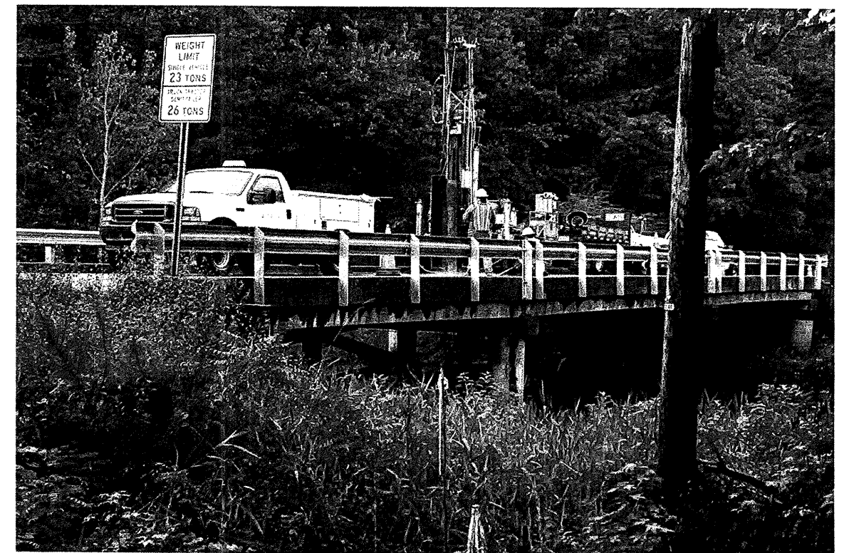
View looking upstation at rig on boring B2.
