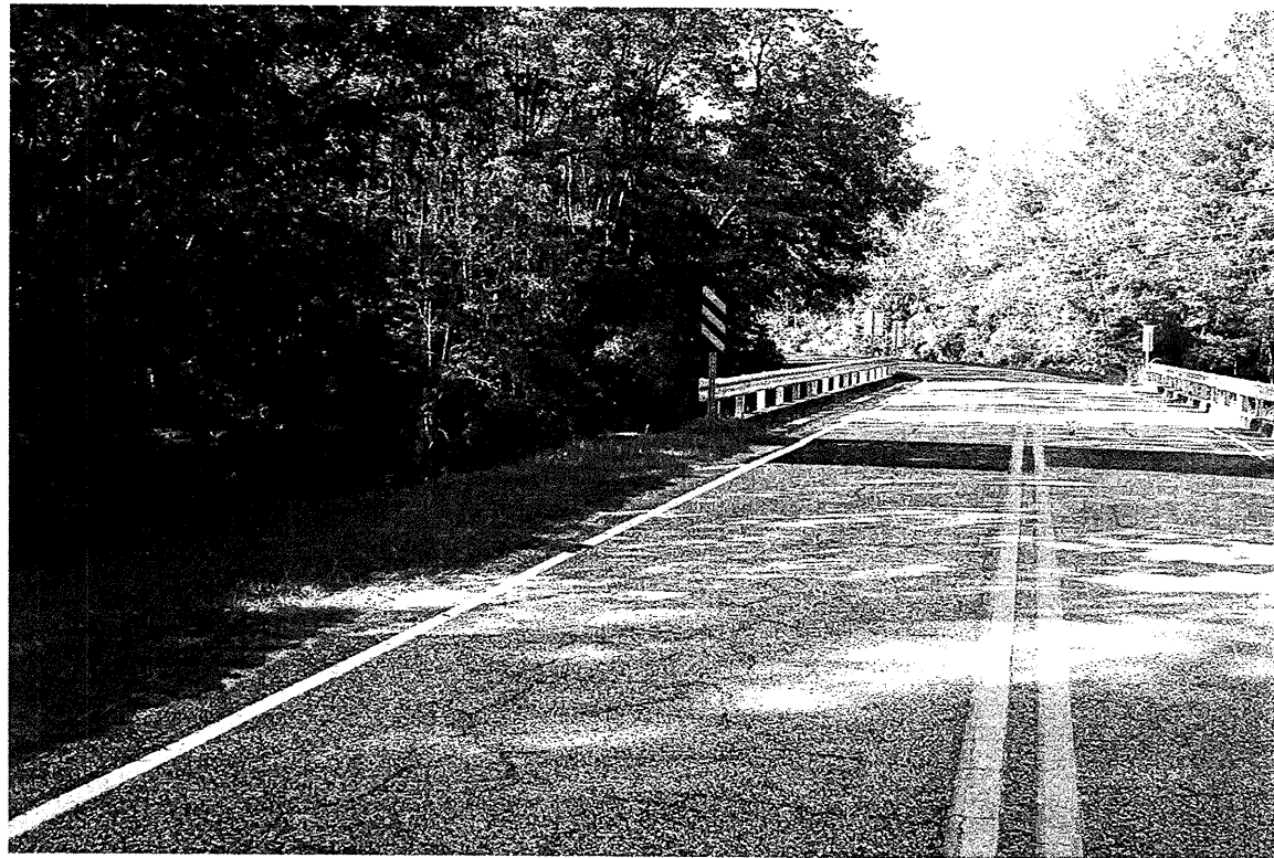
View looking down station along -L- from near End Bent 2.
