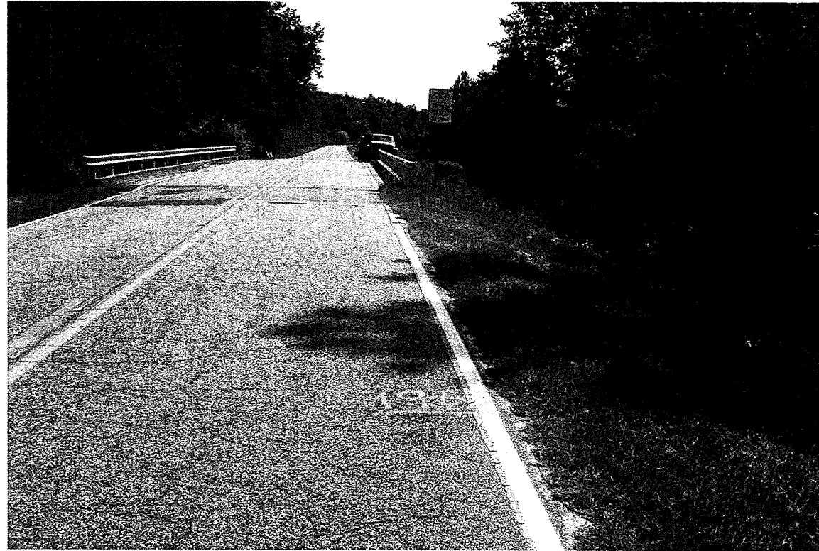
View looking upstation along -L- from Station 19+50.
