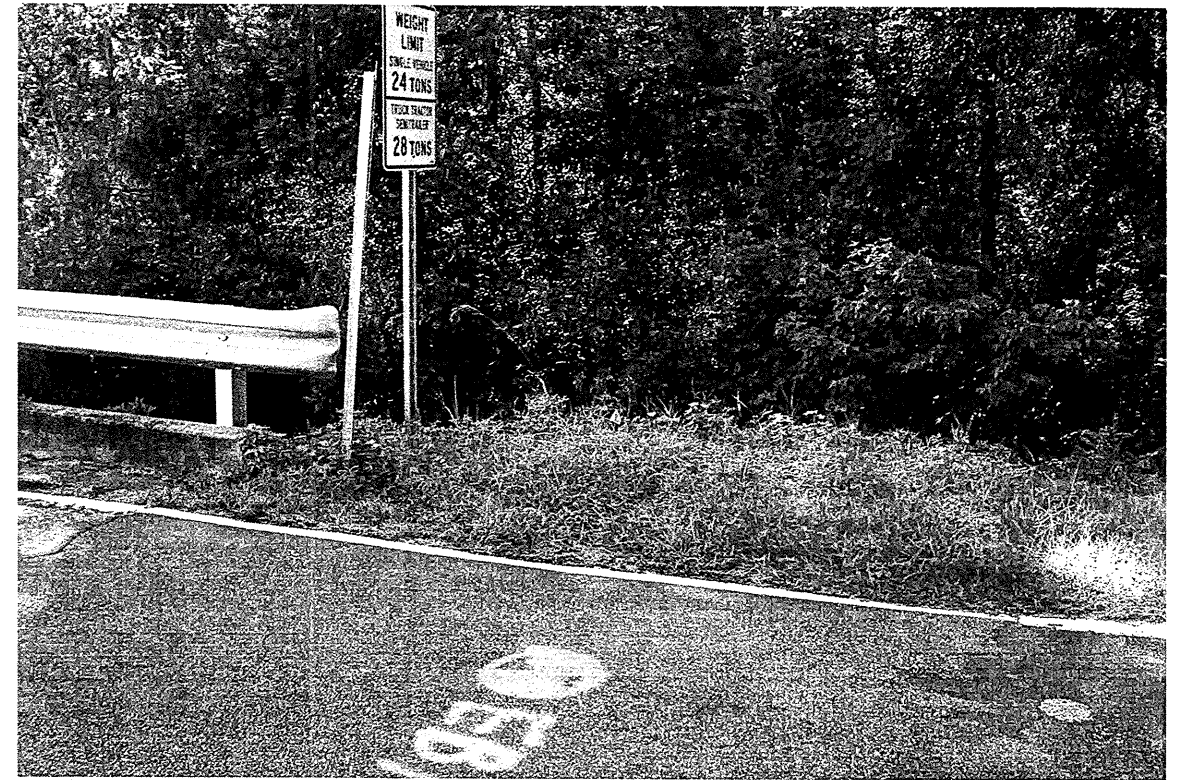
View looking left to right along End Bent 1.
