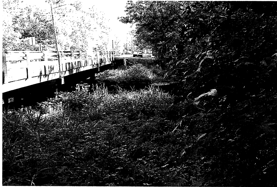
View looking upstation along -L- from near End Bent 1.
