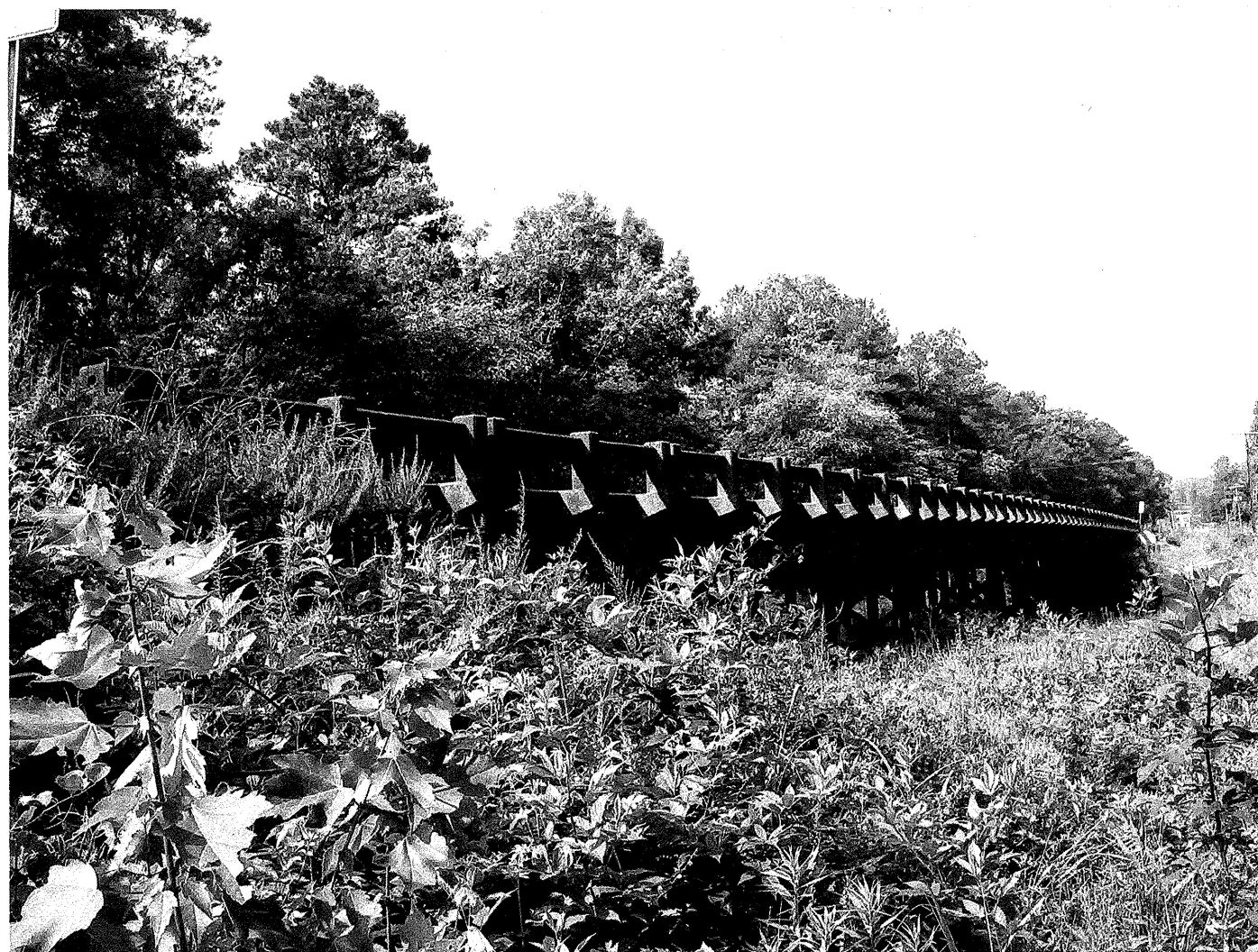
Looking west towards End Bent 1
