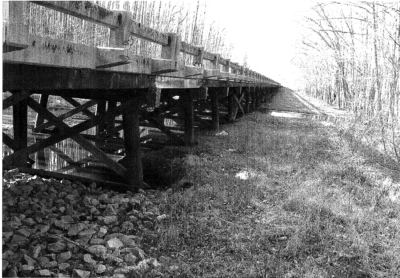
BRIDGE NO. 127 LOOKING SOUTH TOWARDS EB1
