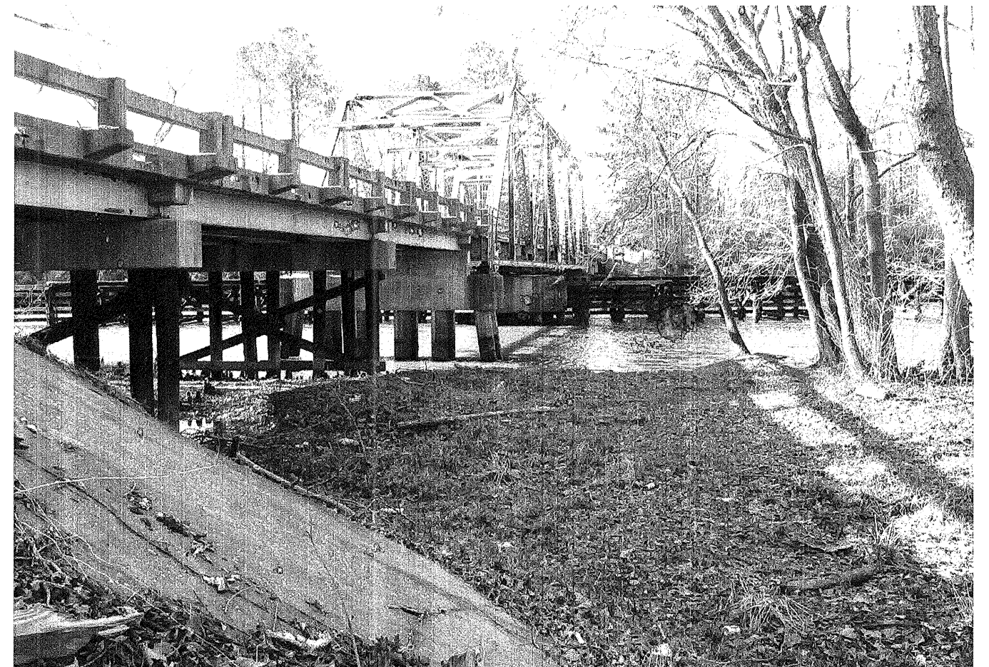
BRIDGE NO. 129 LOOKING SOUTH TOWARDS EB1
