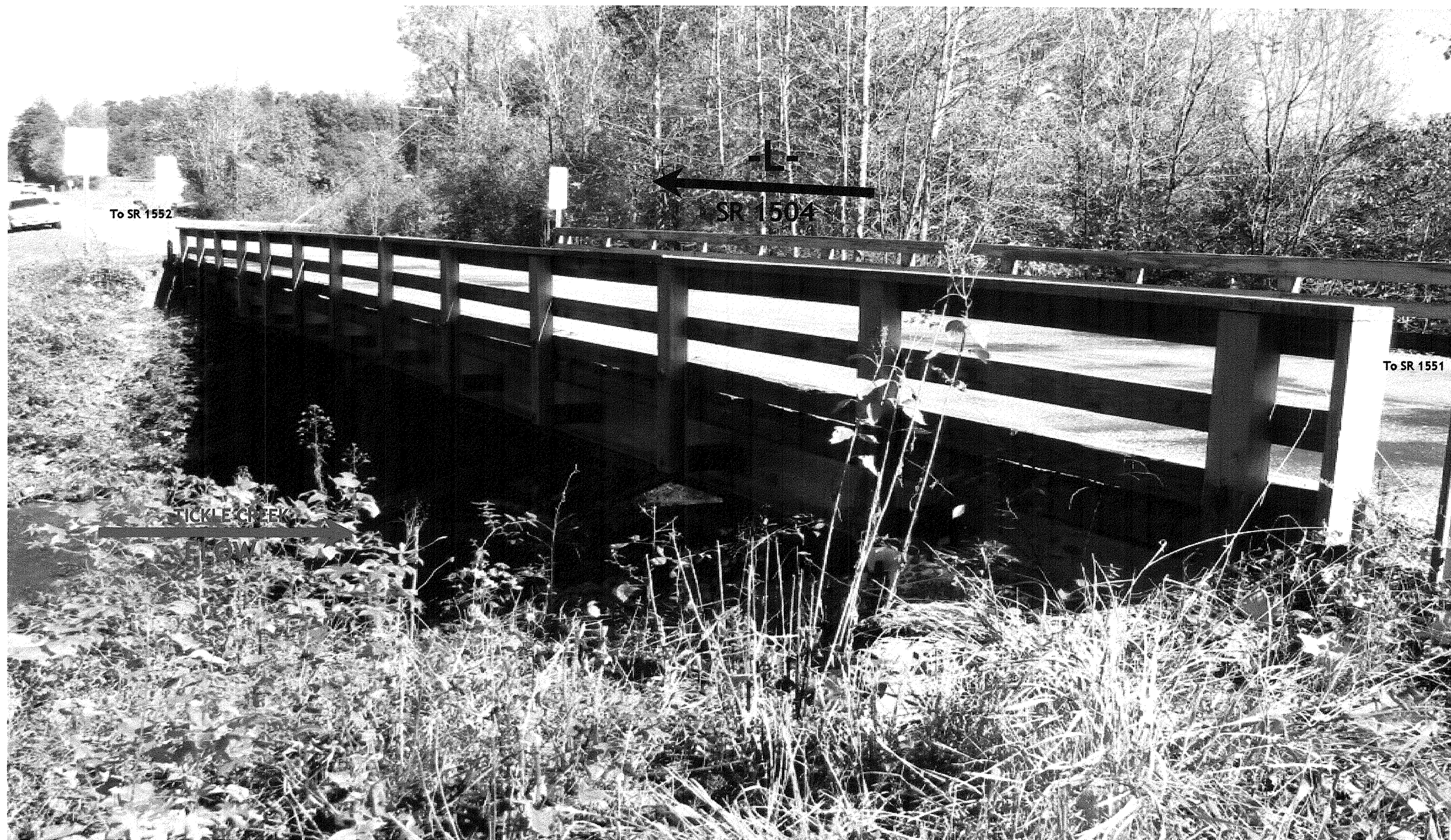
Looking North towards End Bent 2
