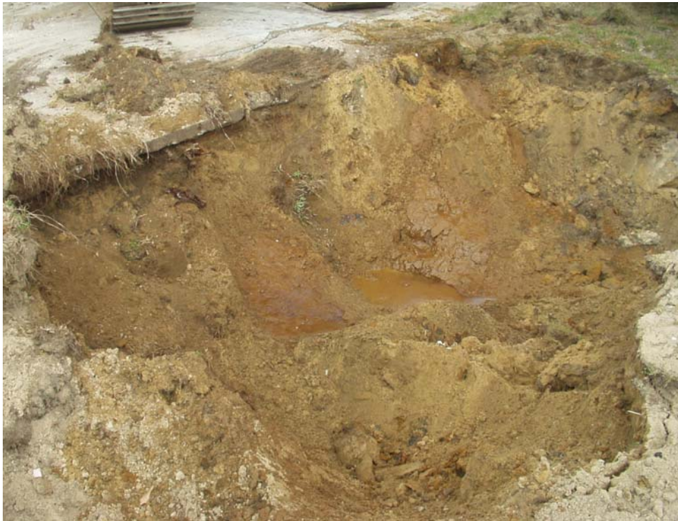
Photograph 4 – Excavation with standing groundwater
