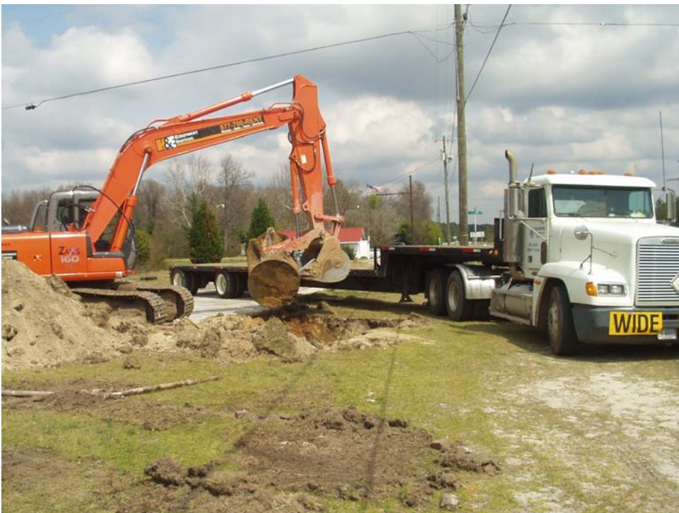
Photograph 2 - Removal of Tank 1
