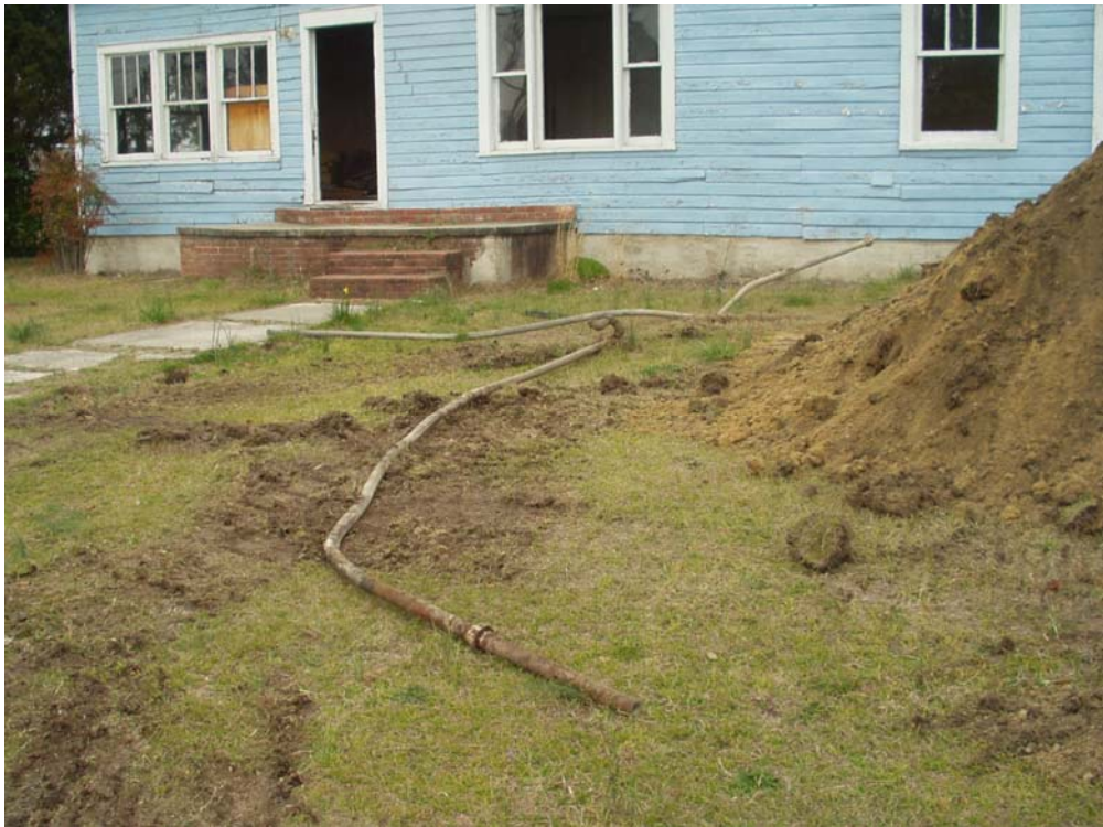
Photograph 6 – Product Lines after removal
