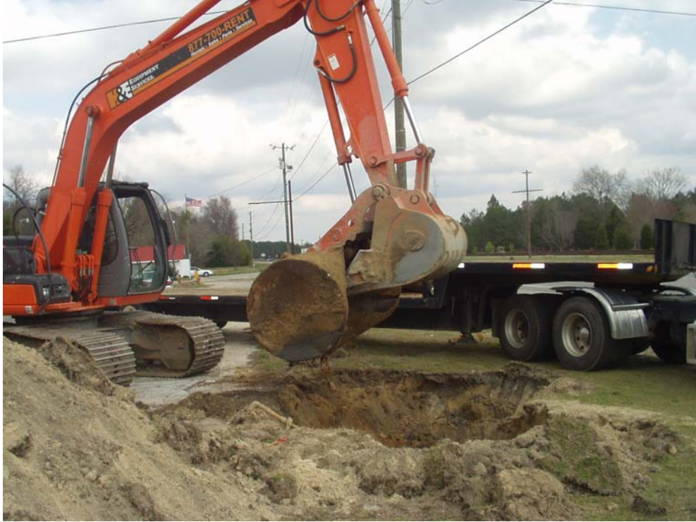
Photograph 3 – Removal of Tank 2
