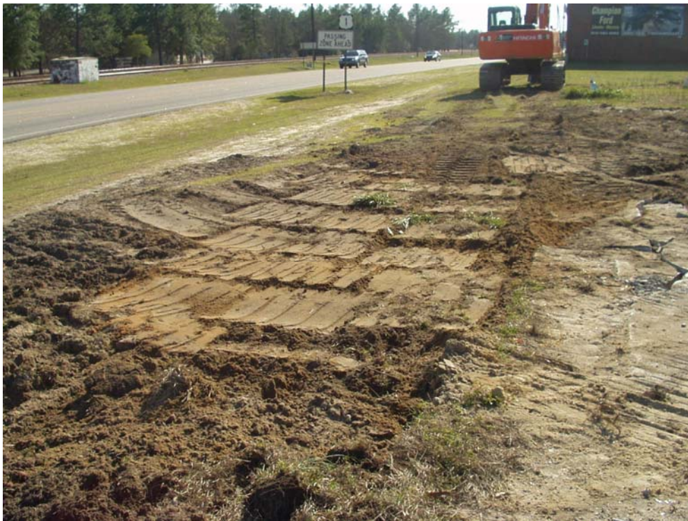
Photograph 8 – Site after backfill
