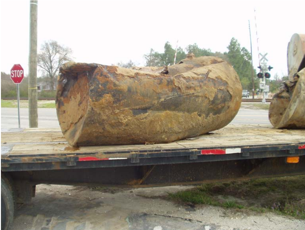
Photograph 7 – Tank 2 after removal
