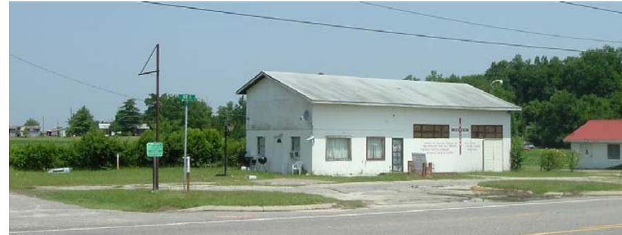
Parcel 51 - Church of Deliverance Property
