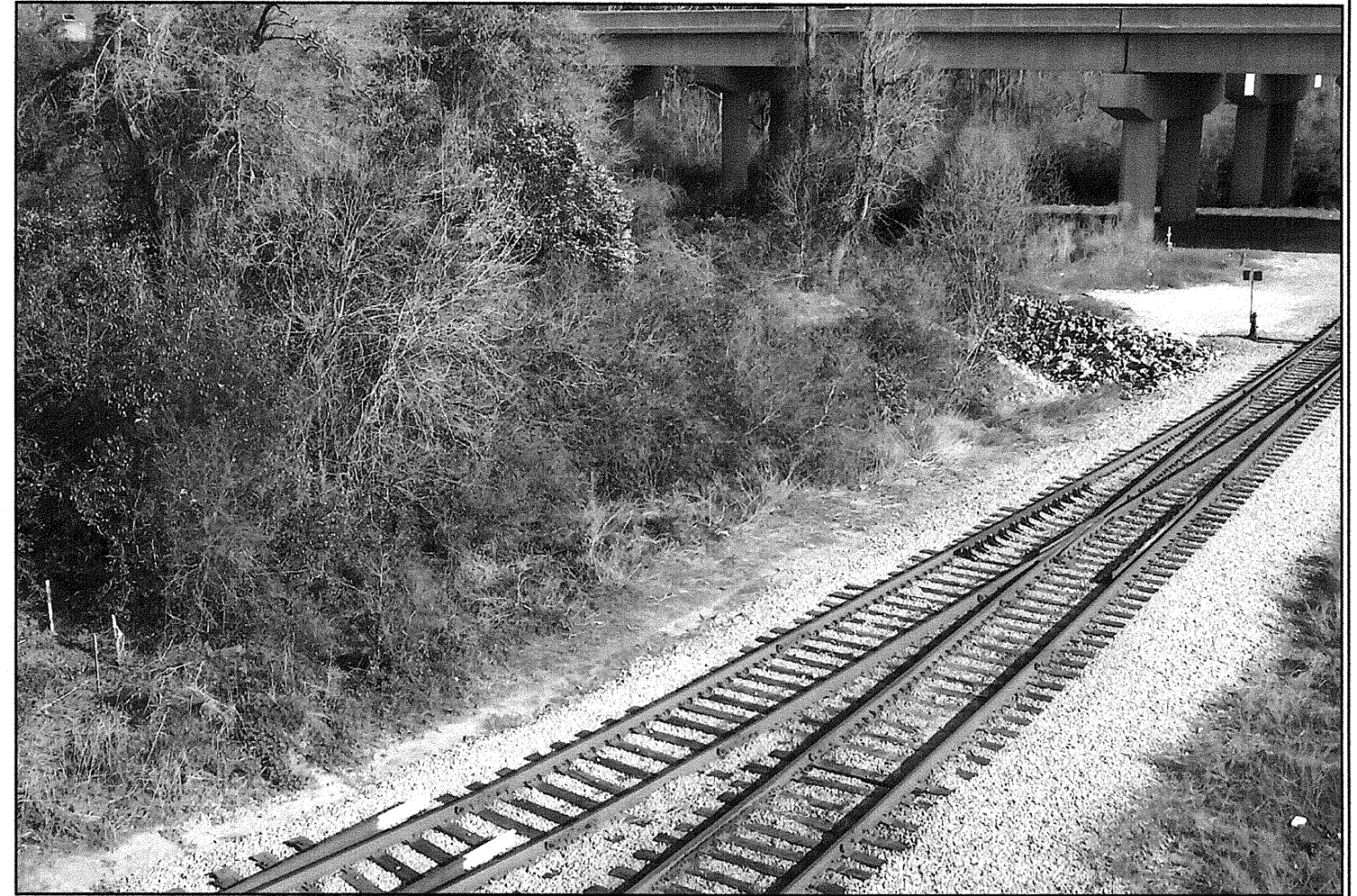
RETAINING WALL 2 (EASTERN SIDE) LOOKING FROM EXISTING BRIDGE 26 TO THE SOUTH.
