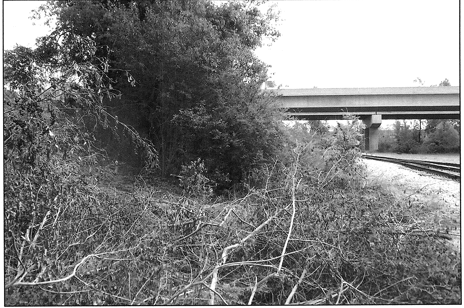
END BENT 2 LOOKING LEFT TO RIGHT.
