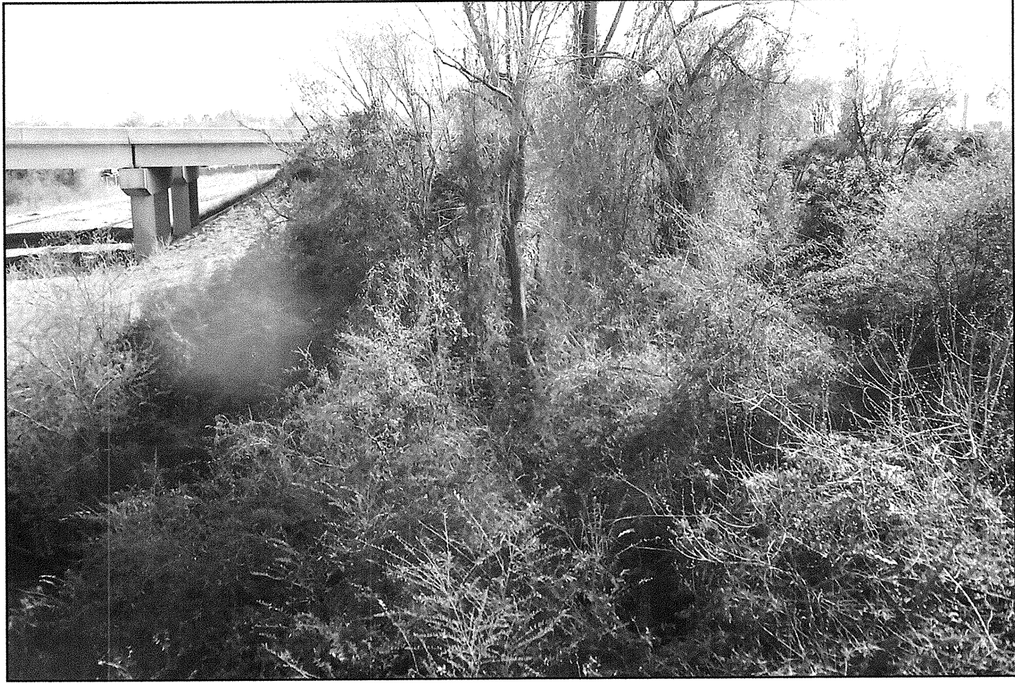
END BENT 1 LOOKING LEFT TO RIGHT.
