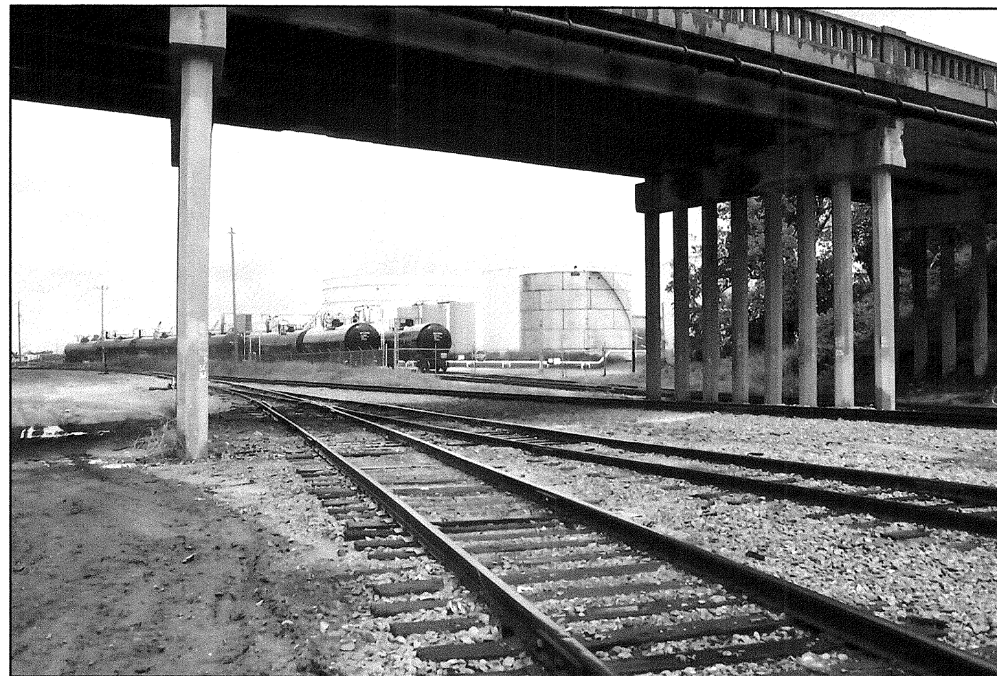
CSXT TRACKS LOOKING NORTH FROM CENTERLINE OF BRIDGE 26.
