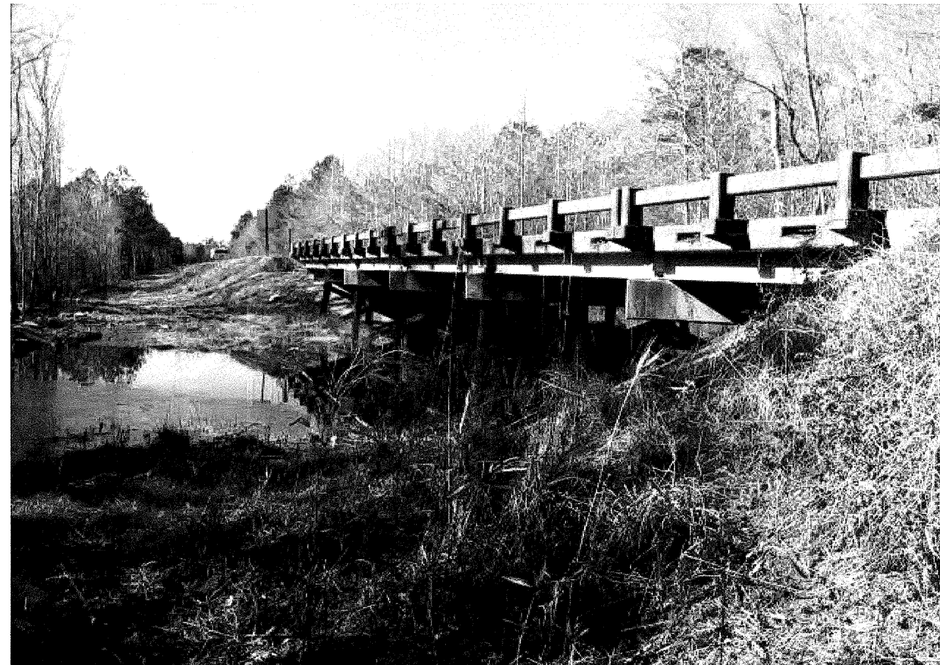
View Looking West Toward End Bent 1
