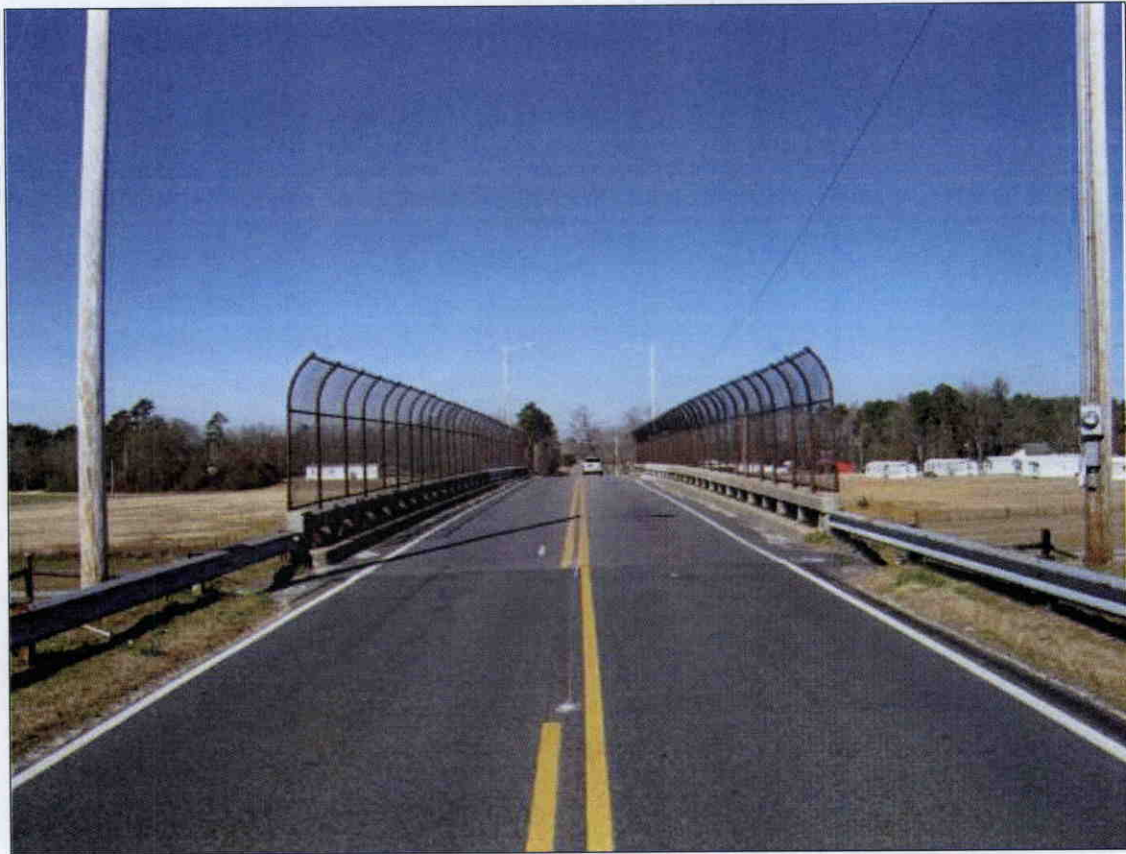
EAST APPROACH LOOKING WEST
