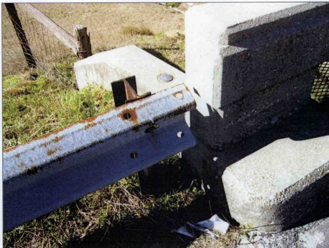
GUARDRAIL ATTACHMENT SOUTHEAST CORNER
