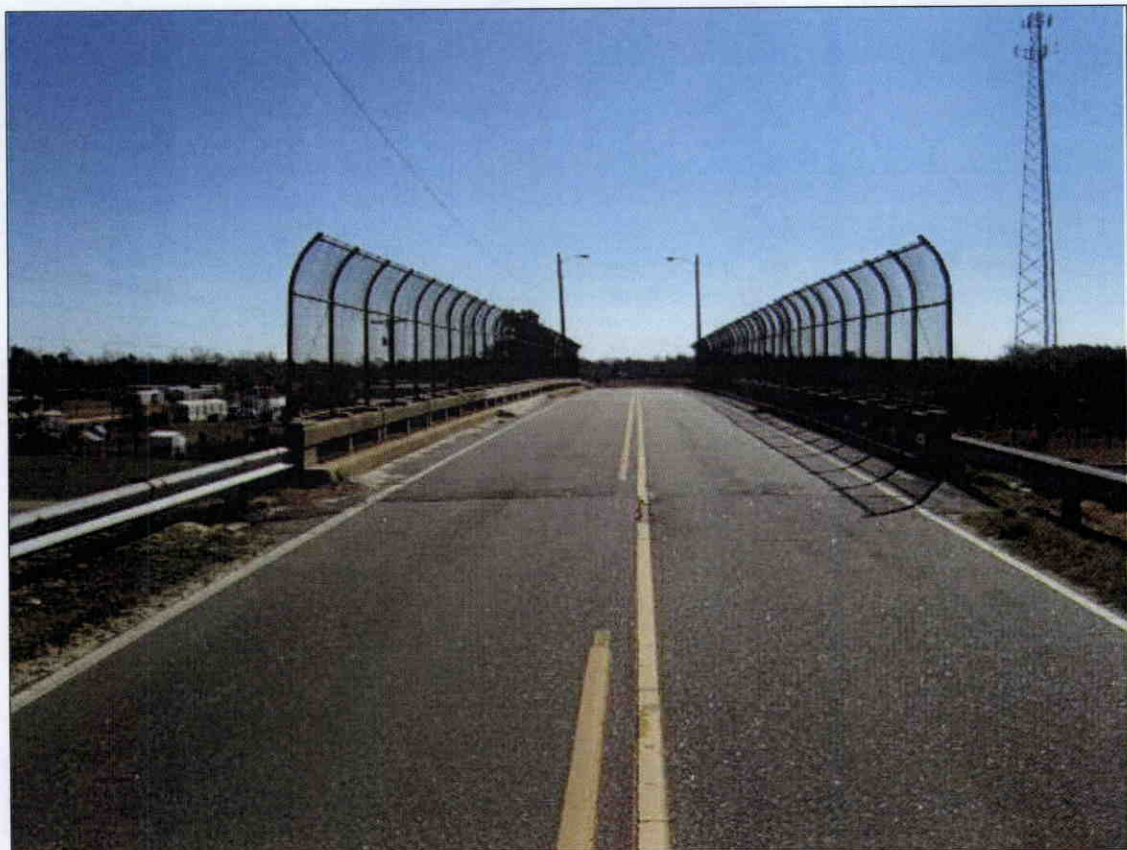
WEST APPROACH LOOKING EAST
