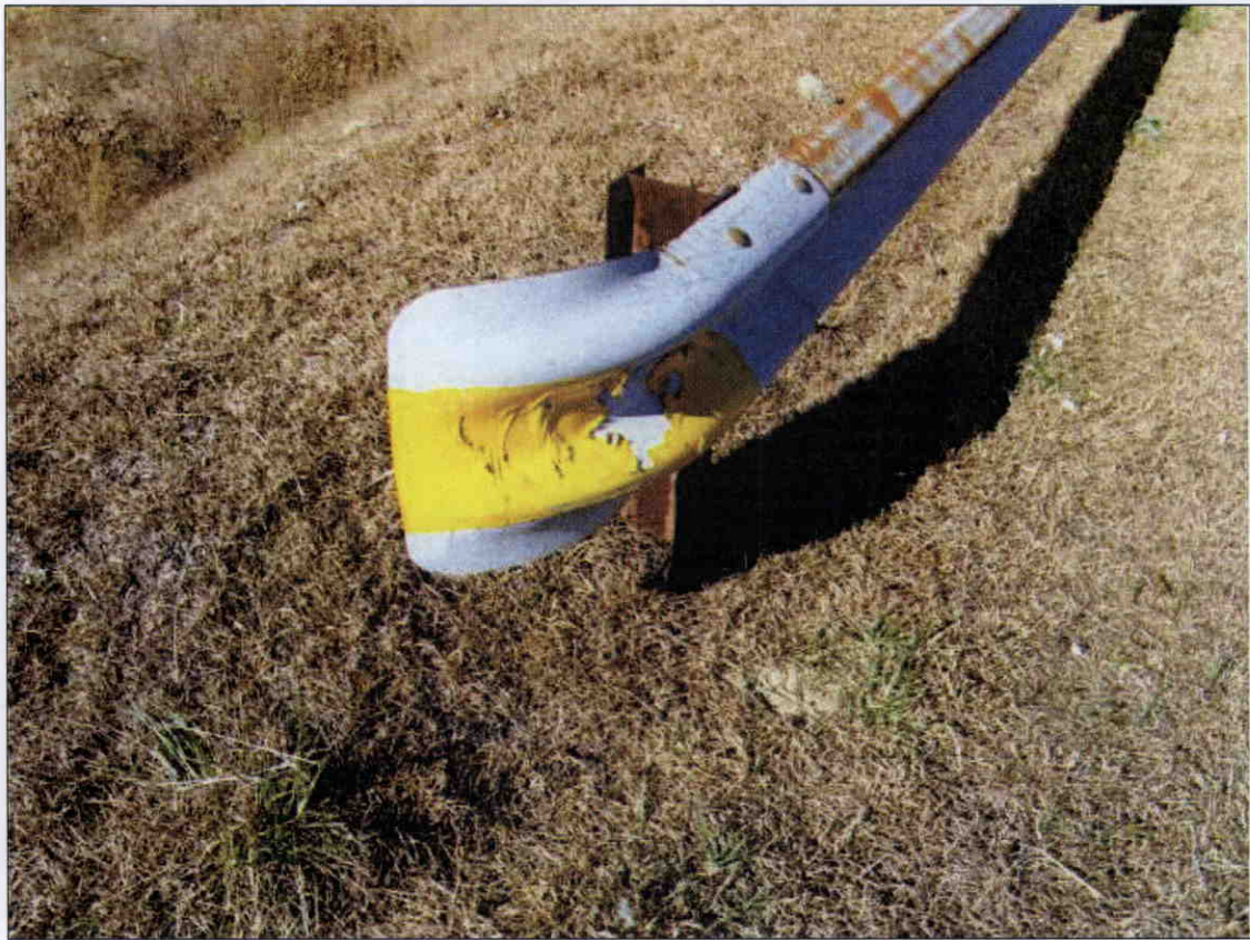
GUARDRAIL TERMINATOR SOUTHEAST CORNER
