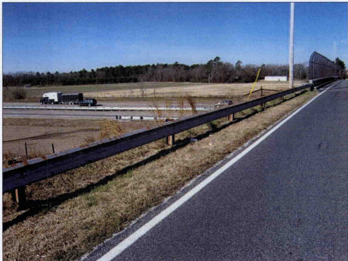
GUARDRAIL POST SPACING 12.5 FT. SOUTHEAST CORNER
