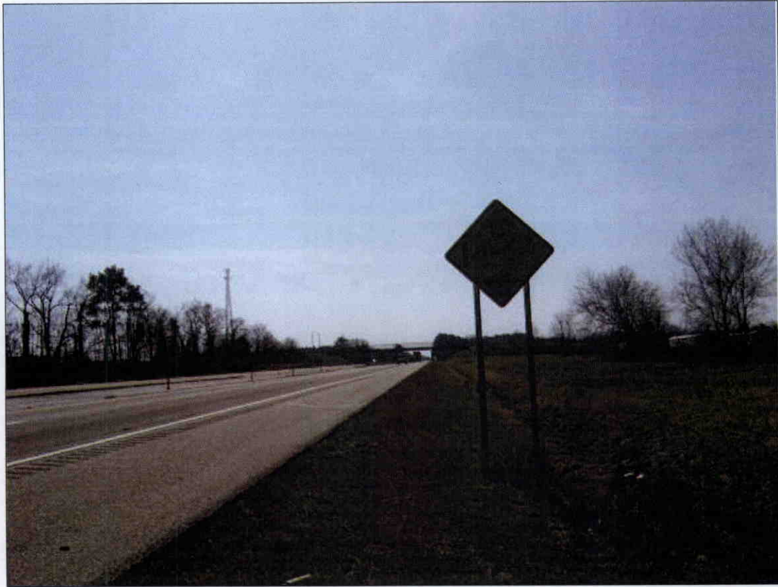
VERTICAL CLEARANCE SIGN 14 FT.-3 IN.ON 95 SB 0.2 MILE NORTH
