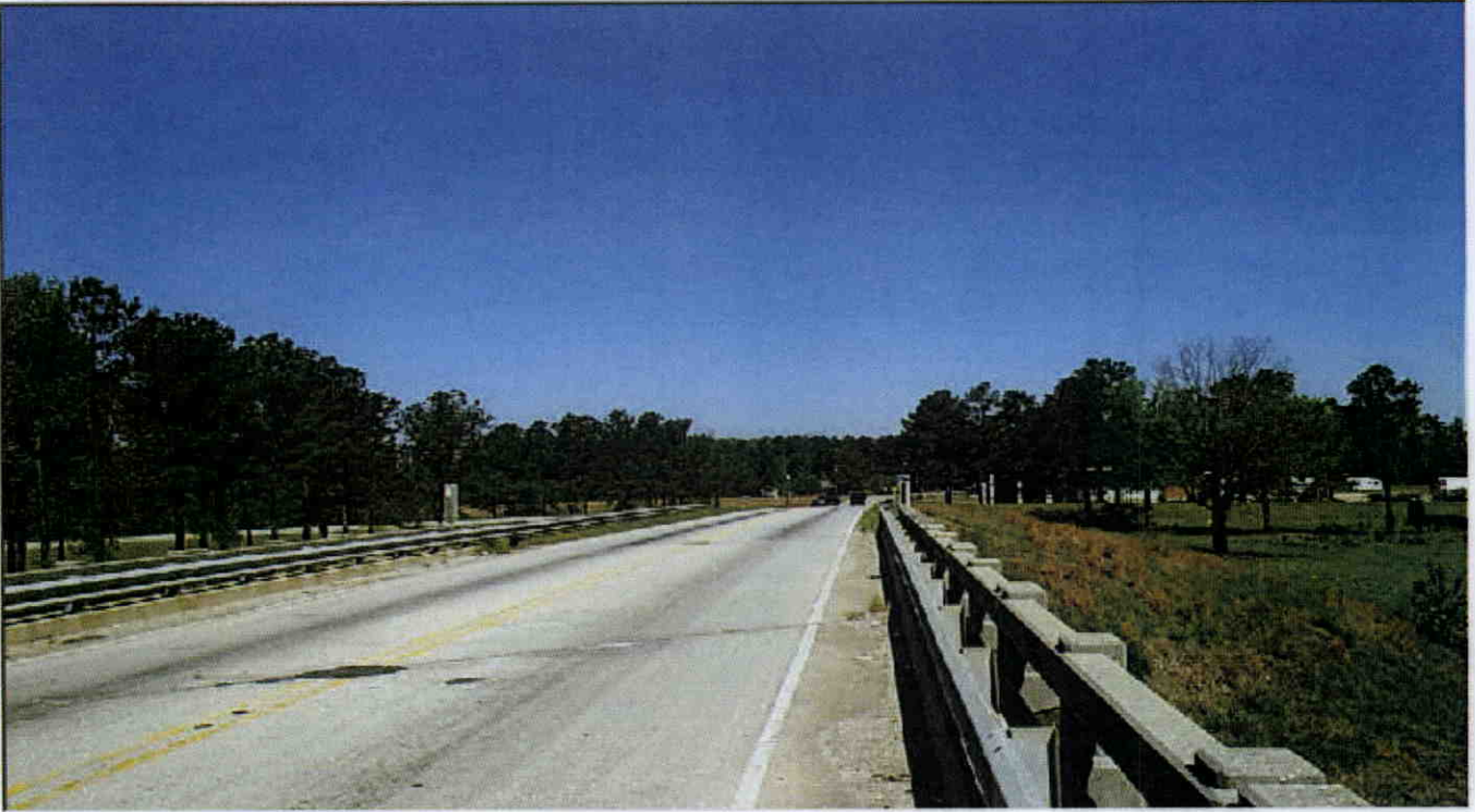
RAMP LOOKING WEST
