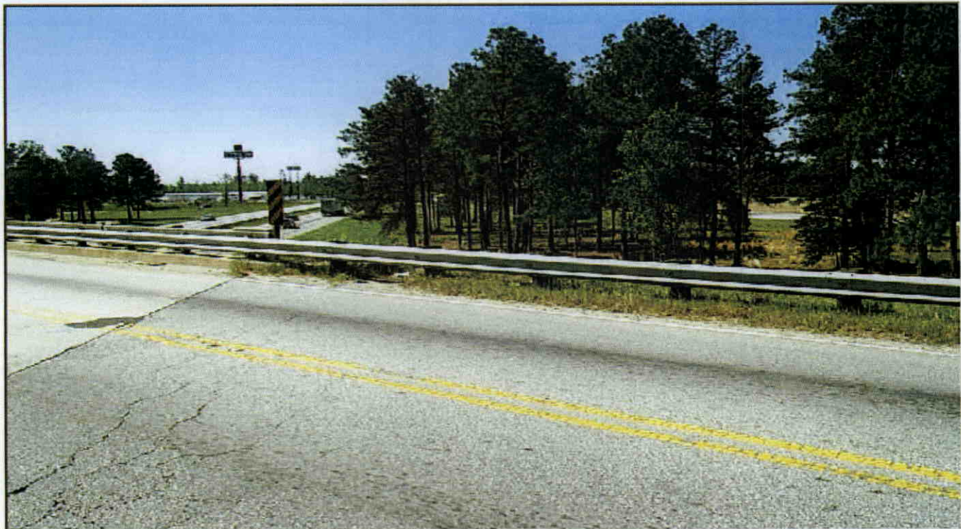
GUARDRAIL POSTS AT ATTACHMENT
