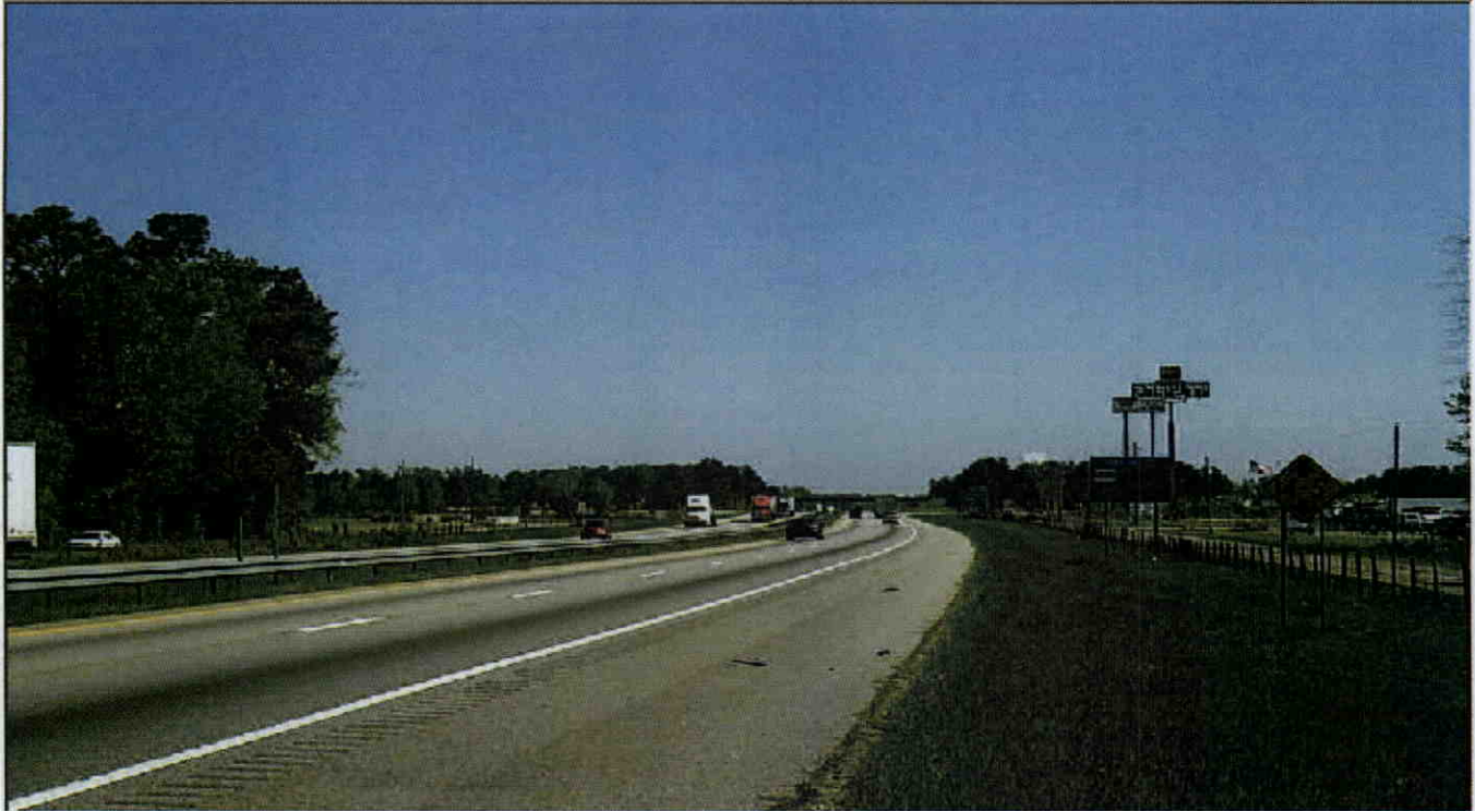
LOW CLEARANCE SIGNS BOTH SIDES NBL 14 FT.5 IN. 0.2 MI. TO BRIDGE.
