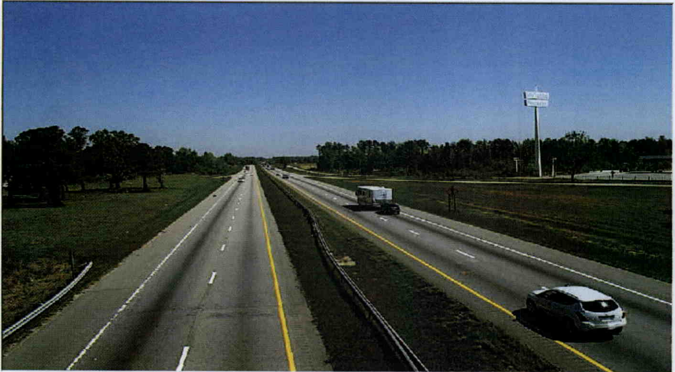
RAMP LOOKING NORTH
