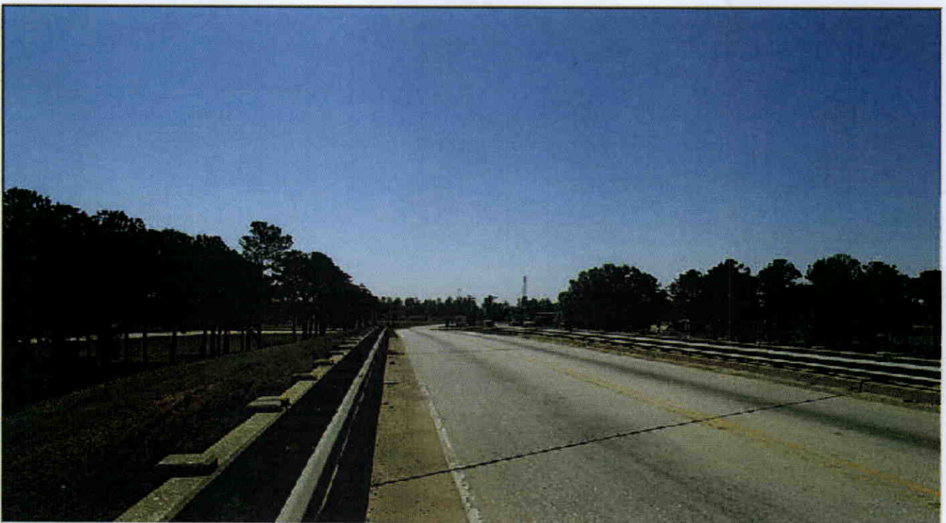
RAMP LOOKING EAST
