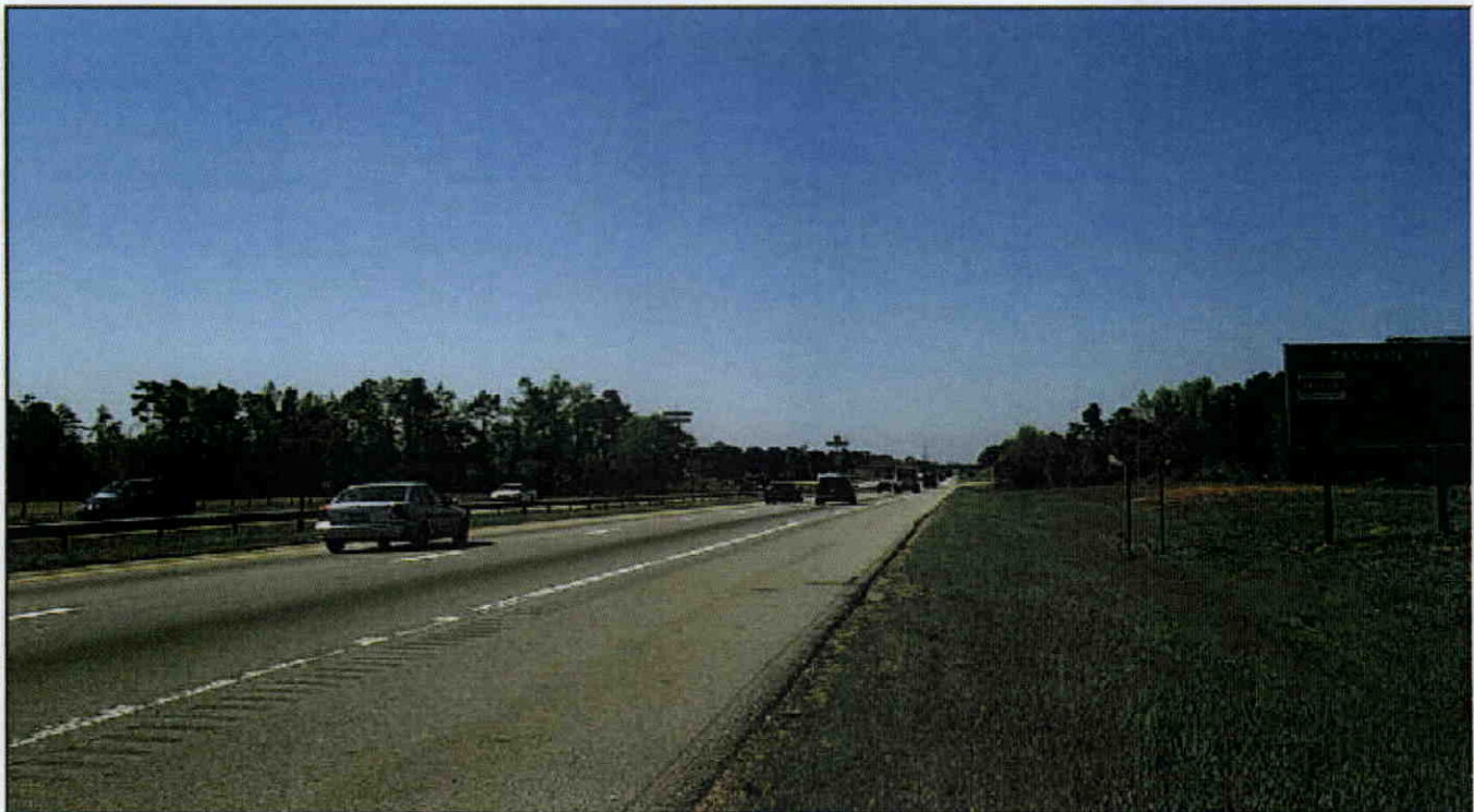
LOW CLEARANCE SIGN SBL BOTH SIDED ROAD 0.2 MI NORTH OF BRIDGE.
