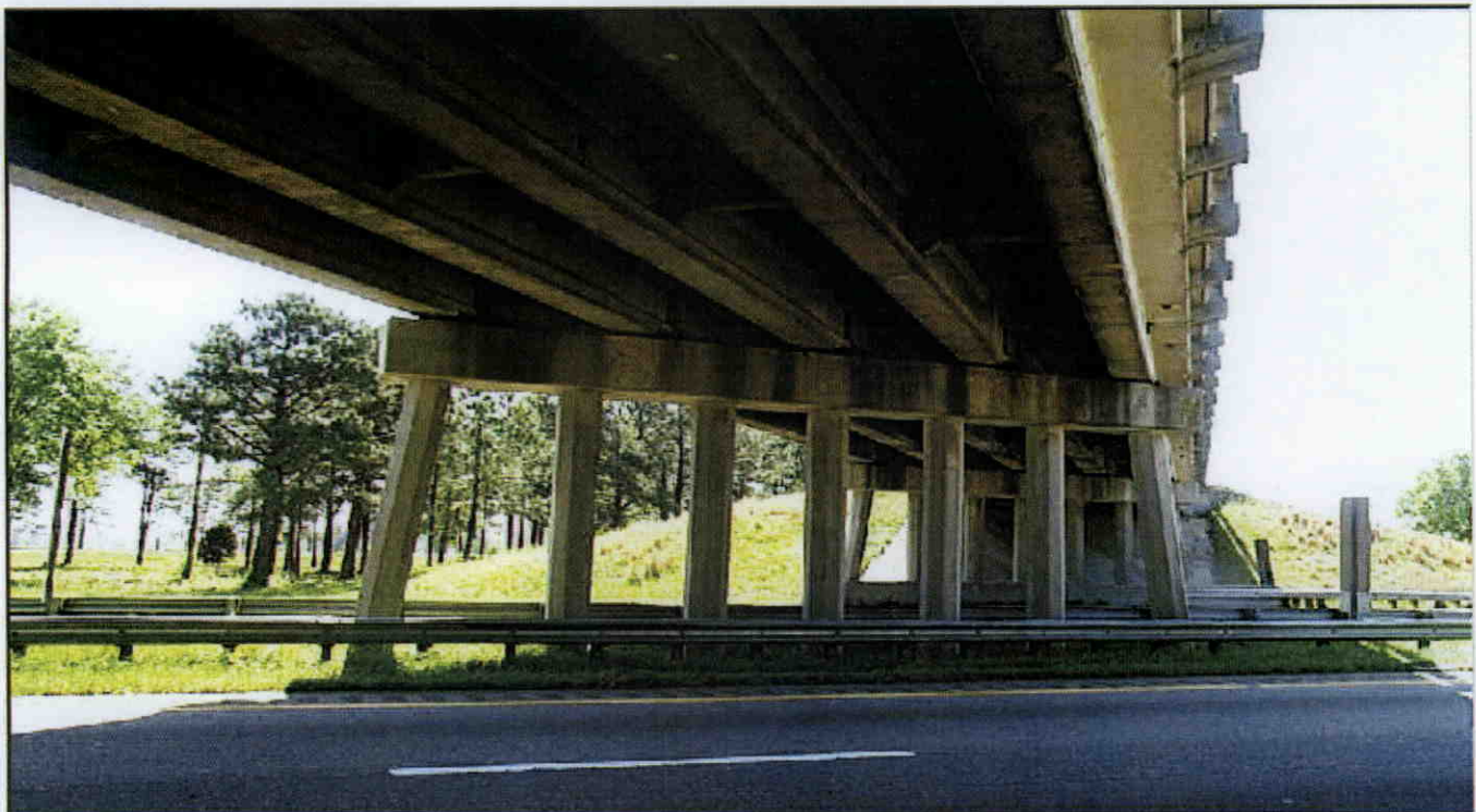
PIER 2, PIERS 1 AND 3 SIMILAR
