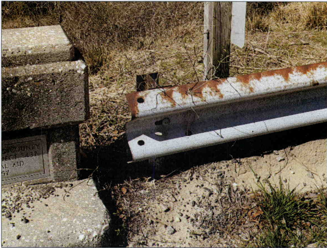
END OF GUARDRAIL AT BRIDGE RAIL
