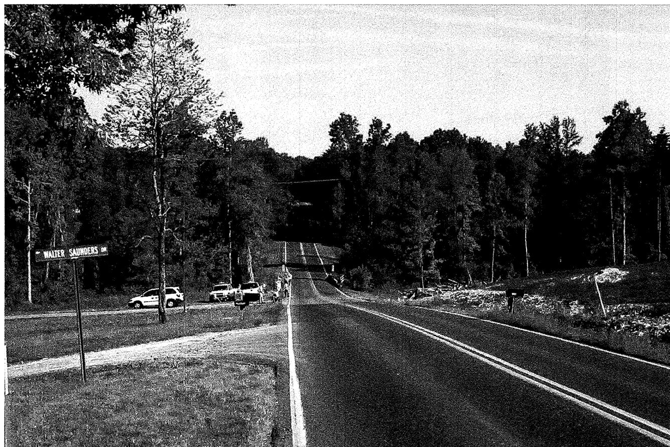
Looking NW (down station)
