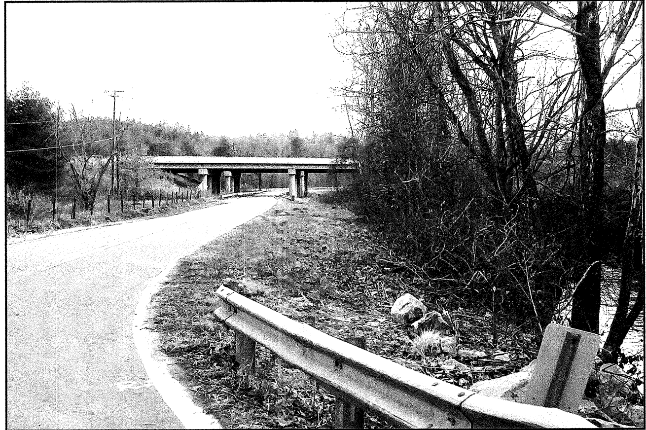
RETAINING WALL PROFILE, LOOKING DOWNSTATION FROM EB1A.
