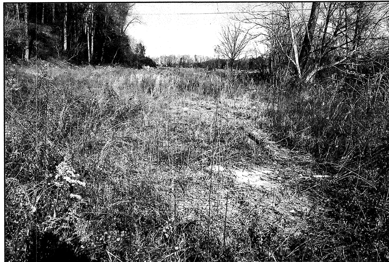
END BENT 2, LOOKING FROM LEFT TO RIGHT.
