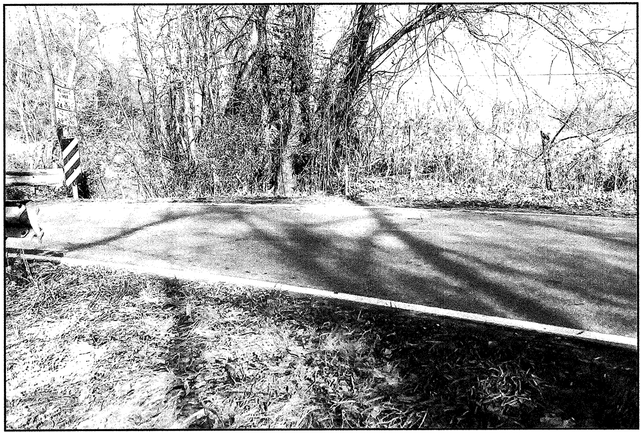
END BENT 1, LOOKING FROM LEFT TO RIGHT.
