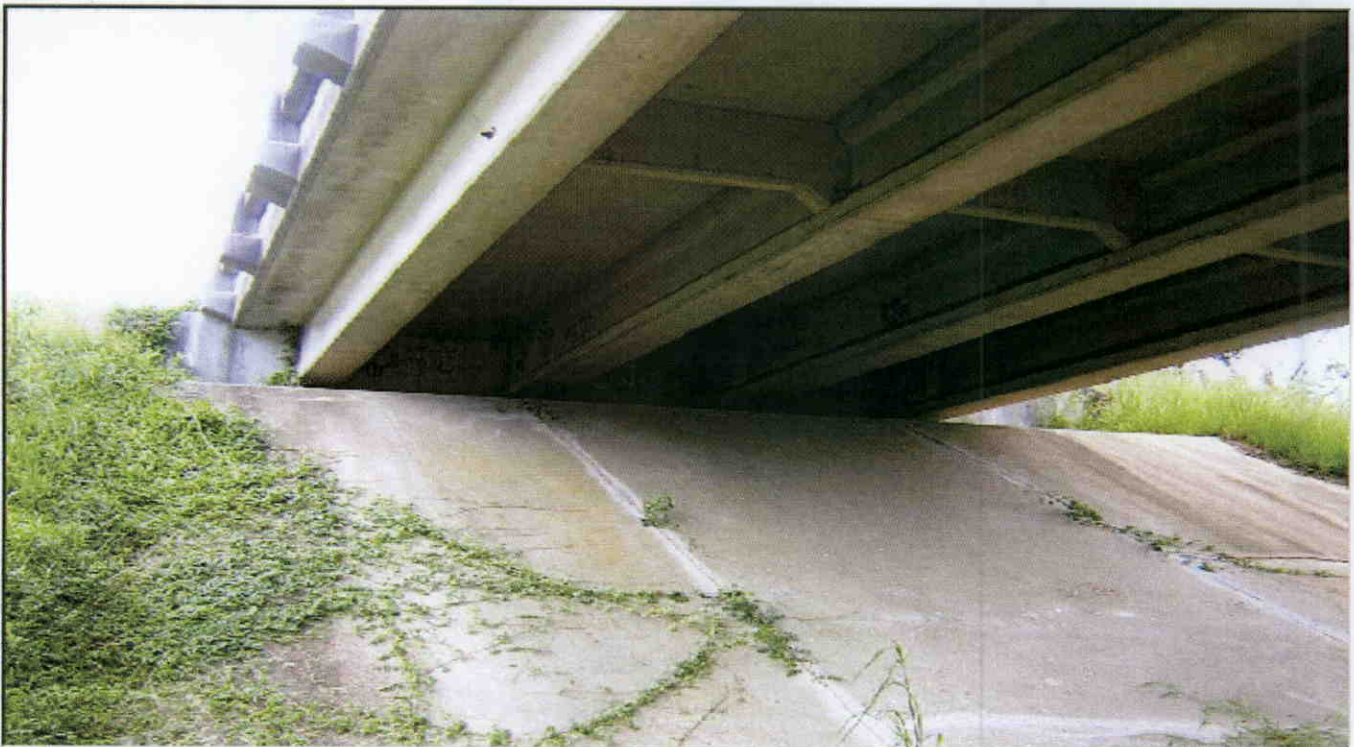
END BENT 2 LOOKING EAST SHORE PROTECTION IN PLACE
