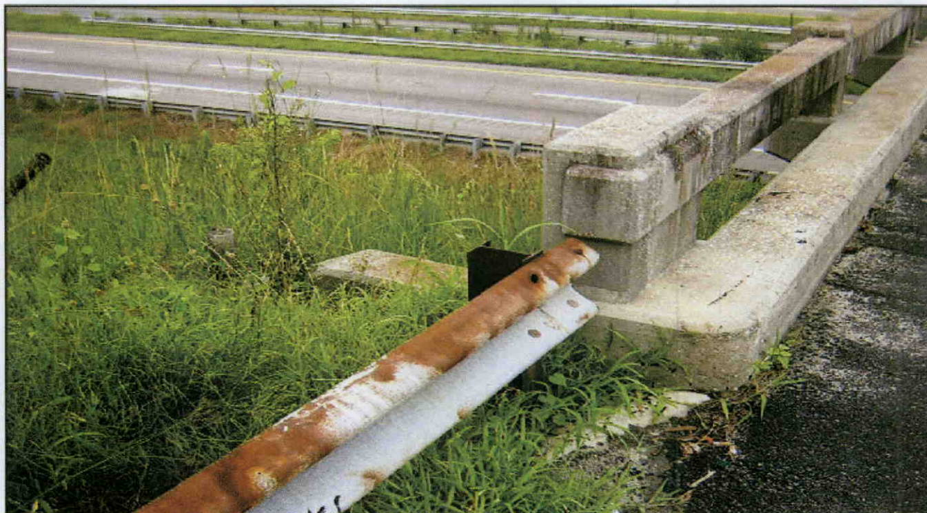
G/R END AT BRIDGE
