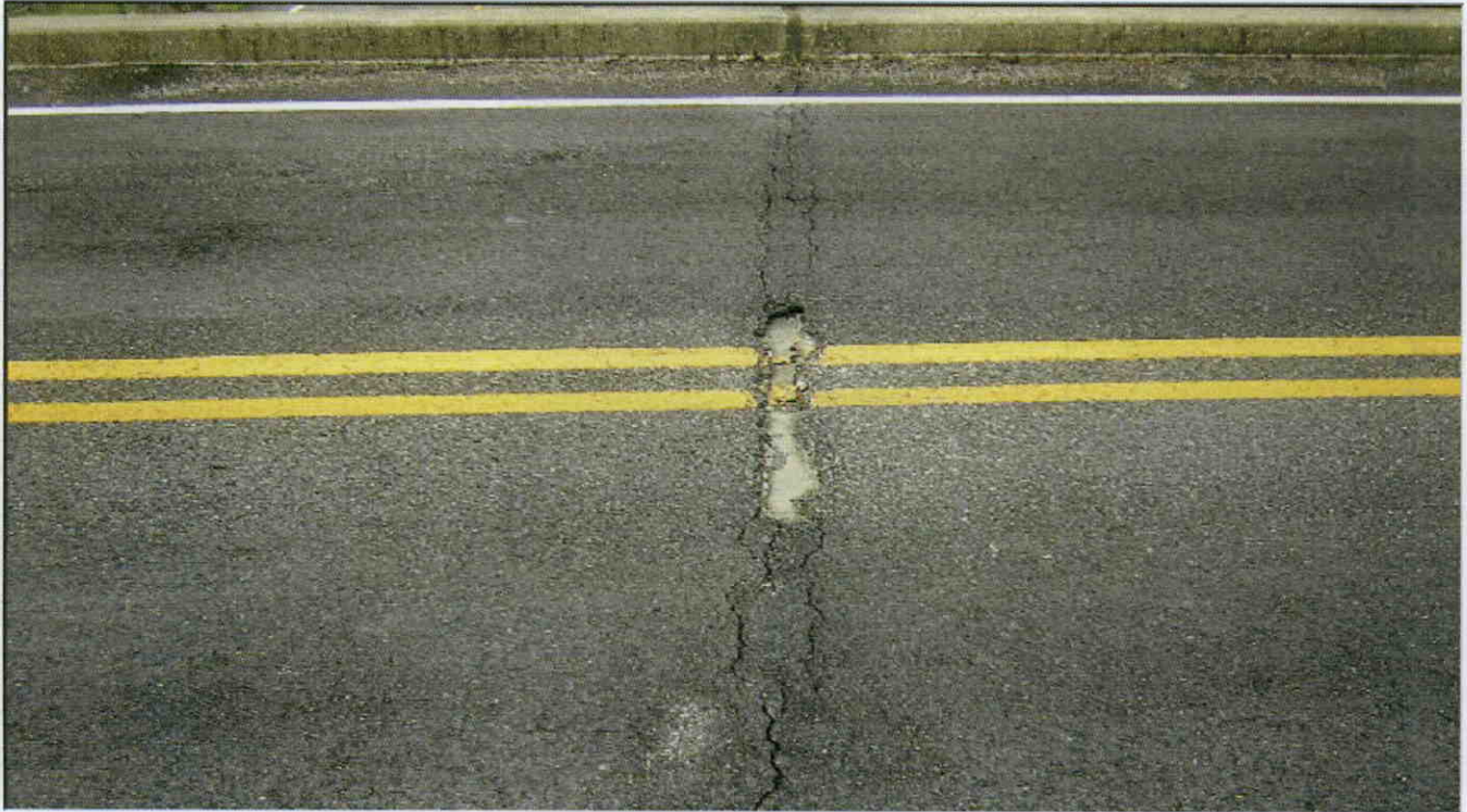
AWS BREAKING UP OVER BENTS
