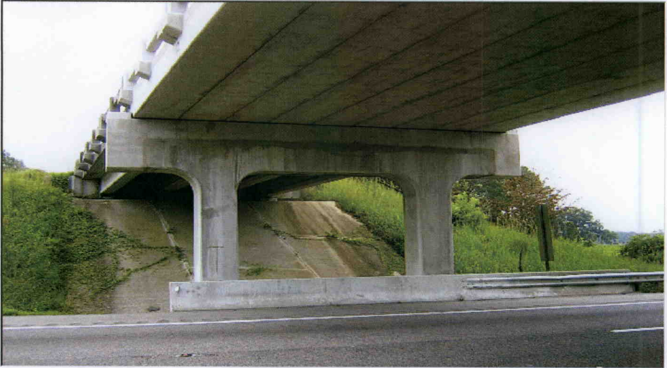
BENT 4 LOOKING EAST BENT 3 SIM.
