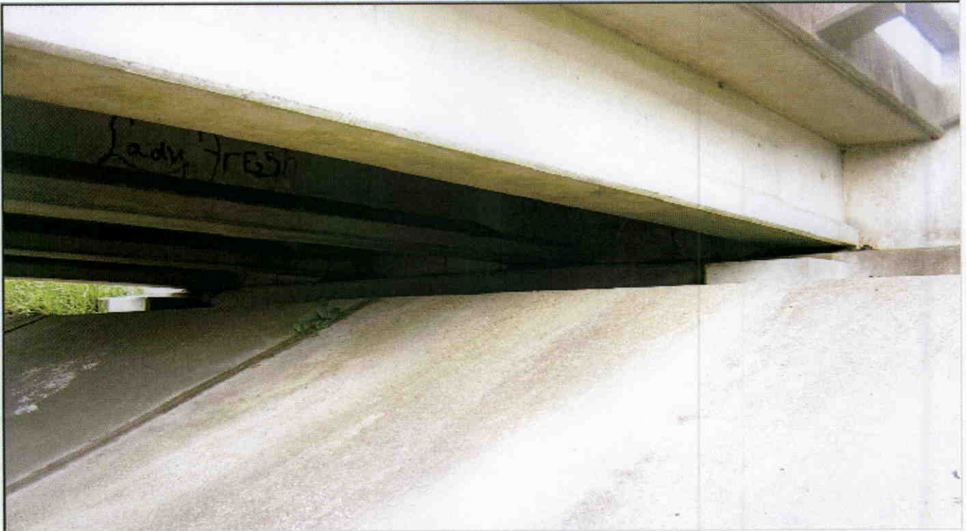
END BENT 1 LOOKING WEST SHORE PROTECTION IN PLACE
