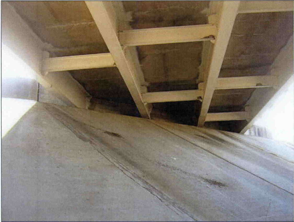
ABUT. 1 LOOKING SOUTH
