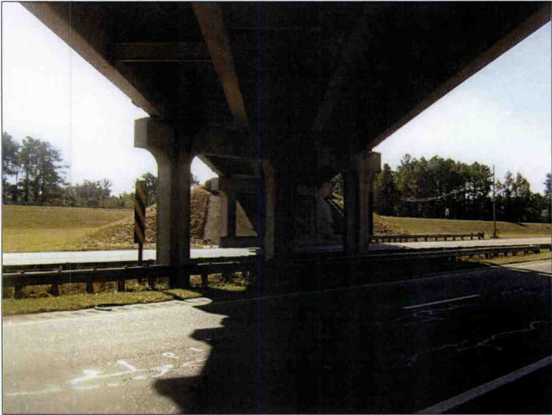
BENT 2 LOOKING SOUTH
