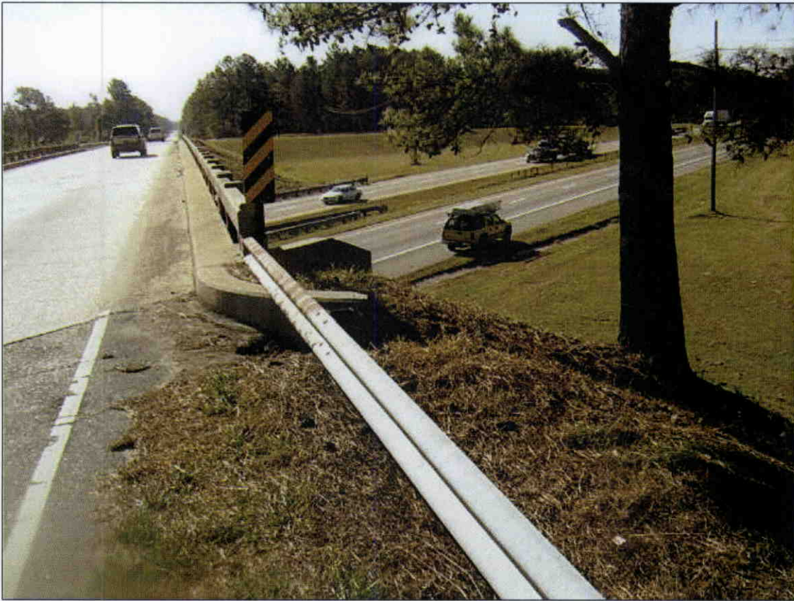
POST SPACING AT BRIDGE
