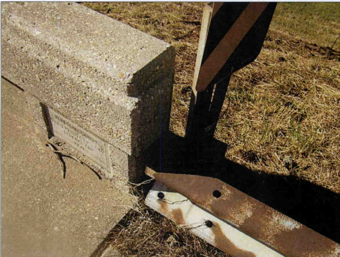
GUARDRAIL END AT BRIDGE
