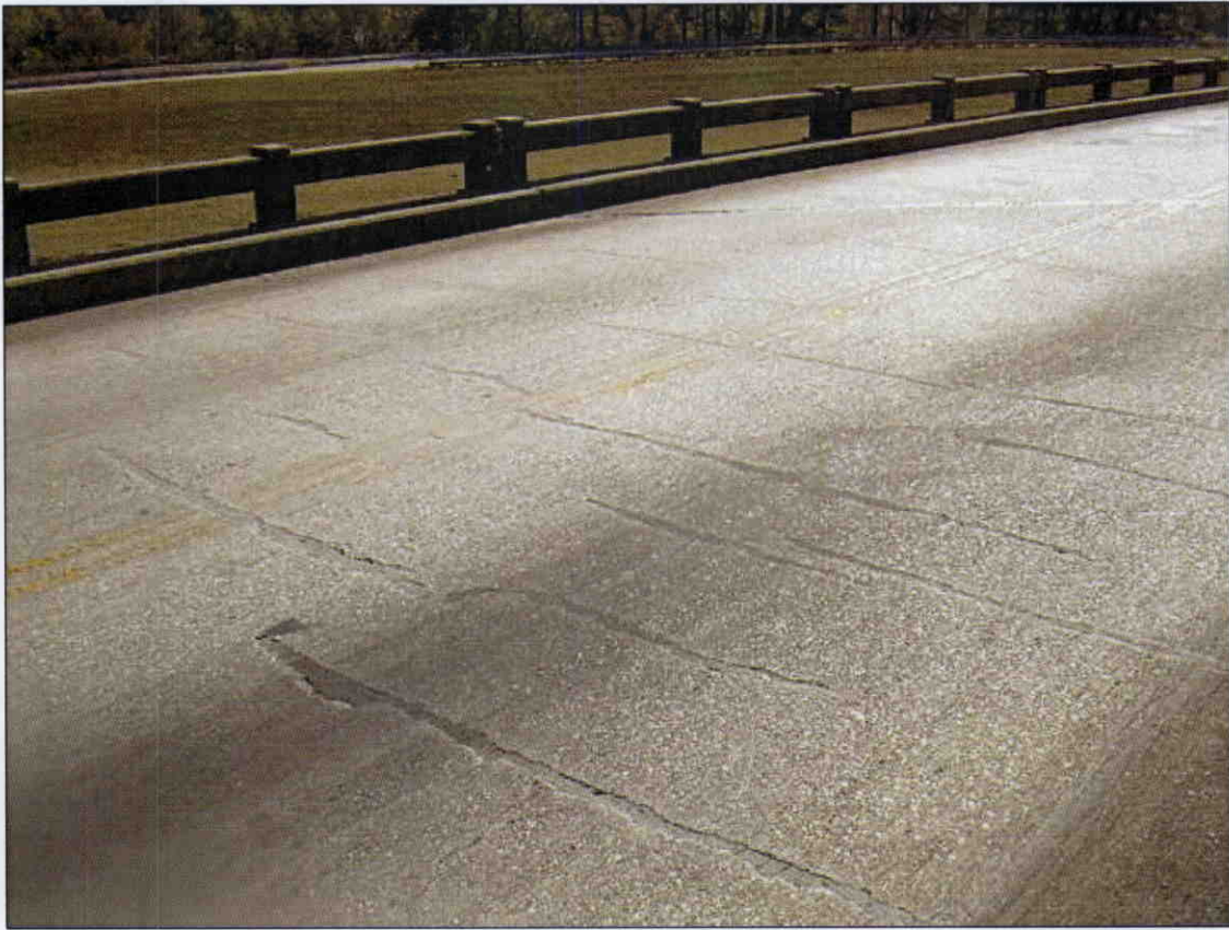
CRACKS IN TOP SIDE OF DECK SEALED
