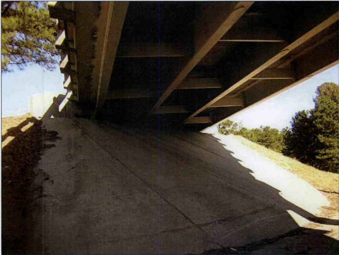
ABUT. 2 LOOKING NORTH
