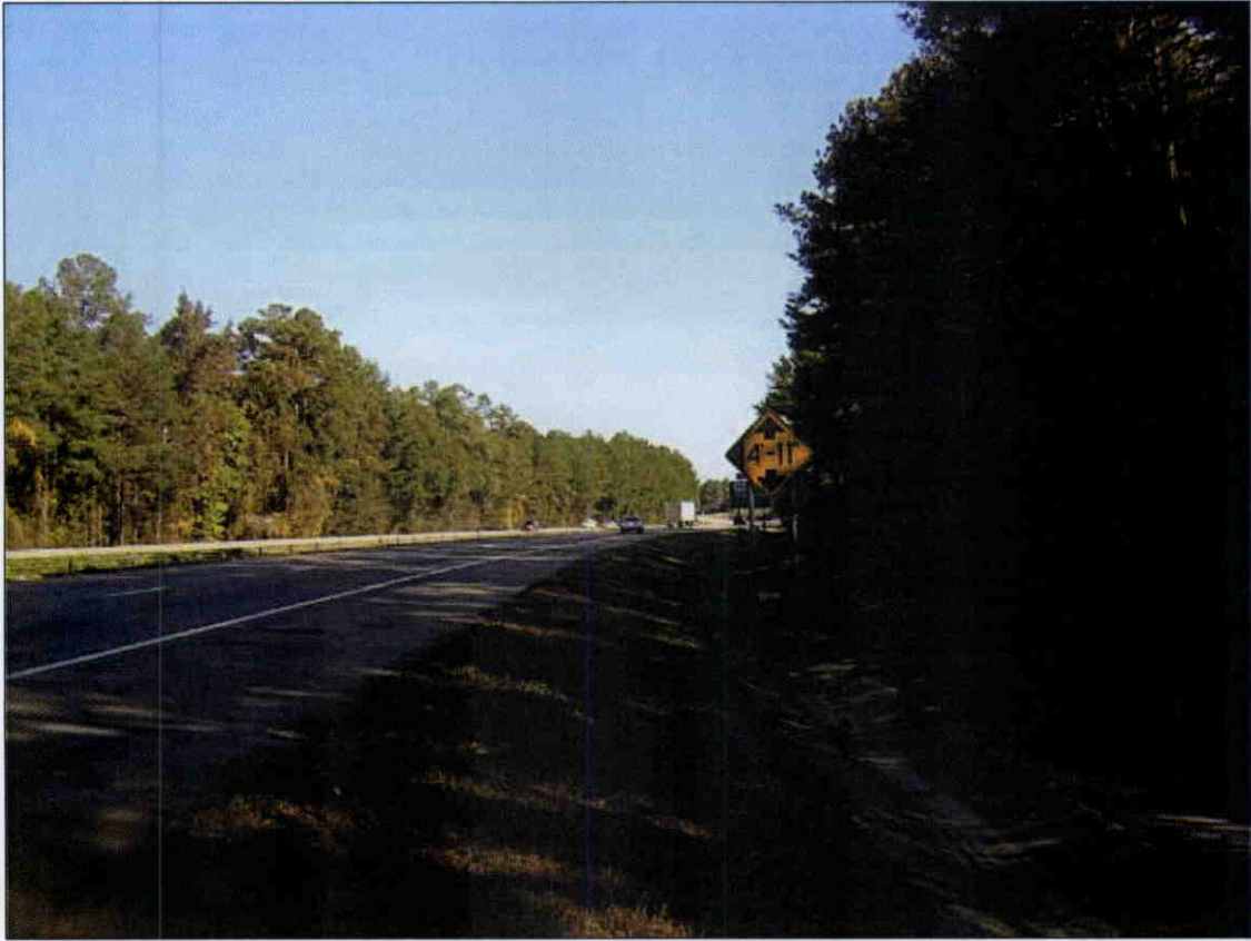
VERTICAL CLR. SIGN 14 FT.11 IN. SOUTH OF BRIDGE
