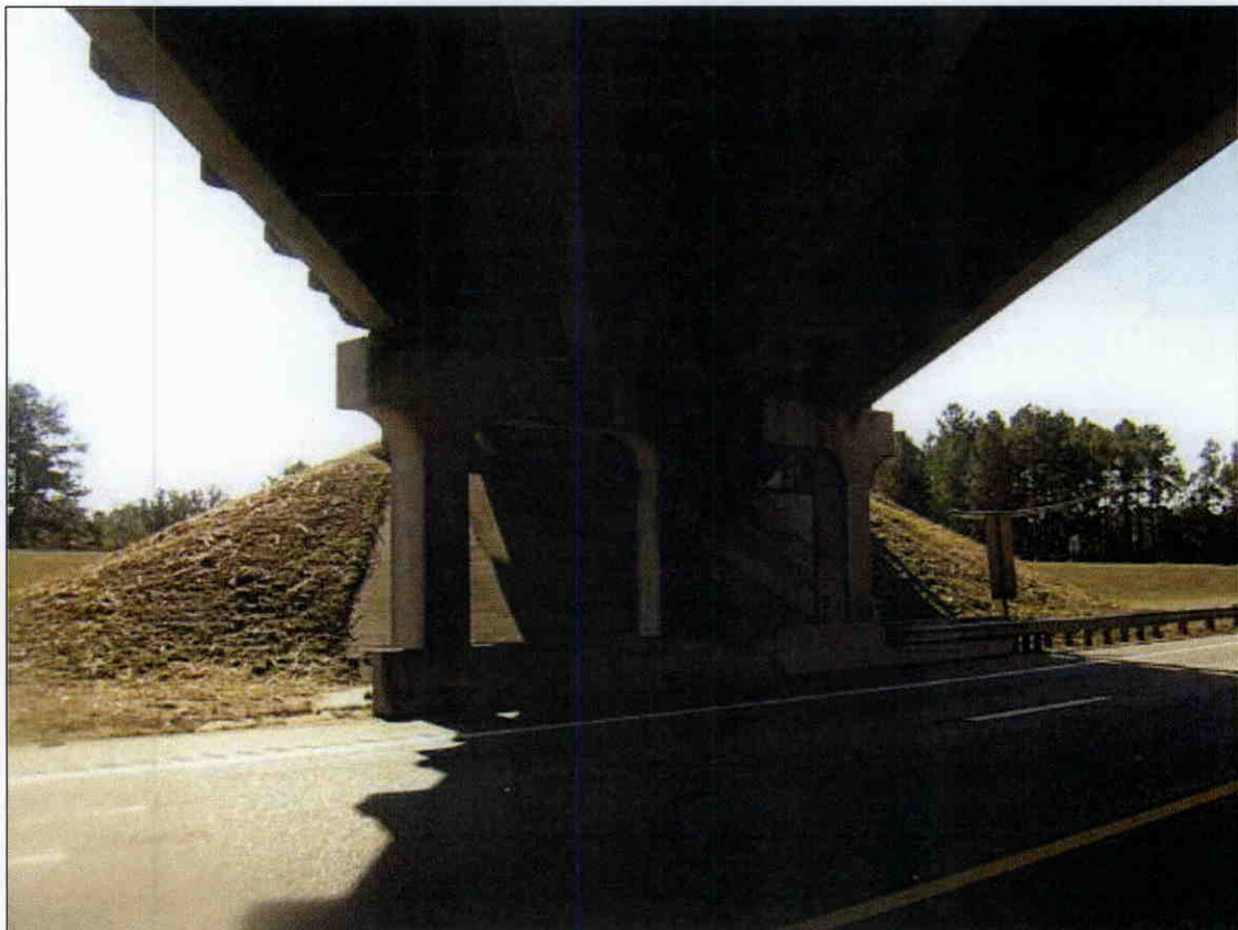
PIER 1 LOOKING SOUTH PIER 3 SIM.
