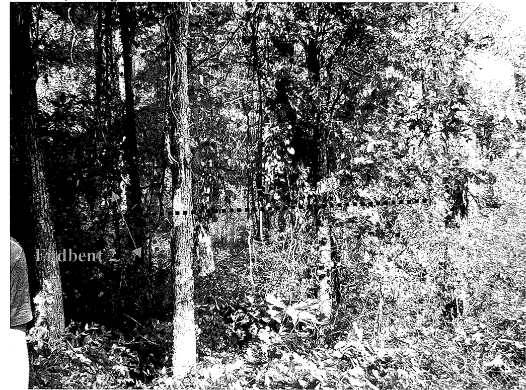
Endbent 2, Looking From B to A, (Northerly)
