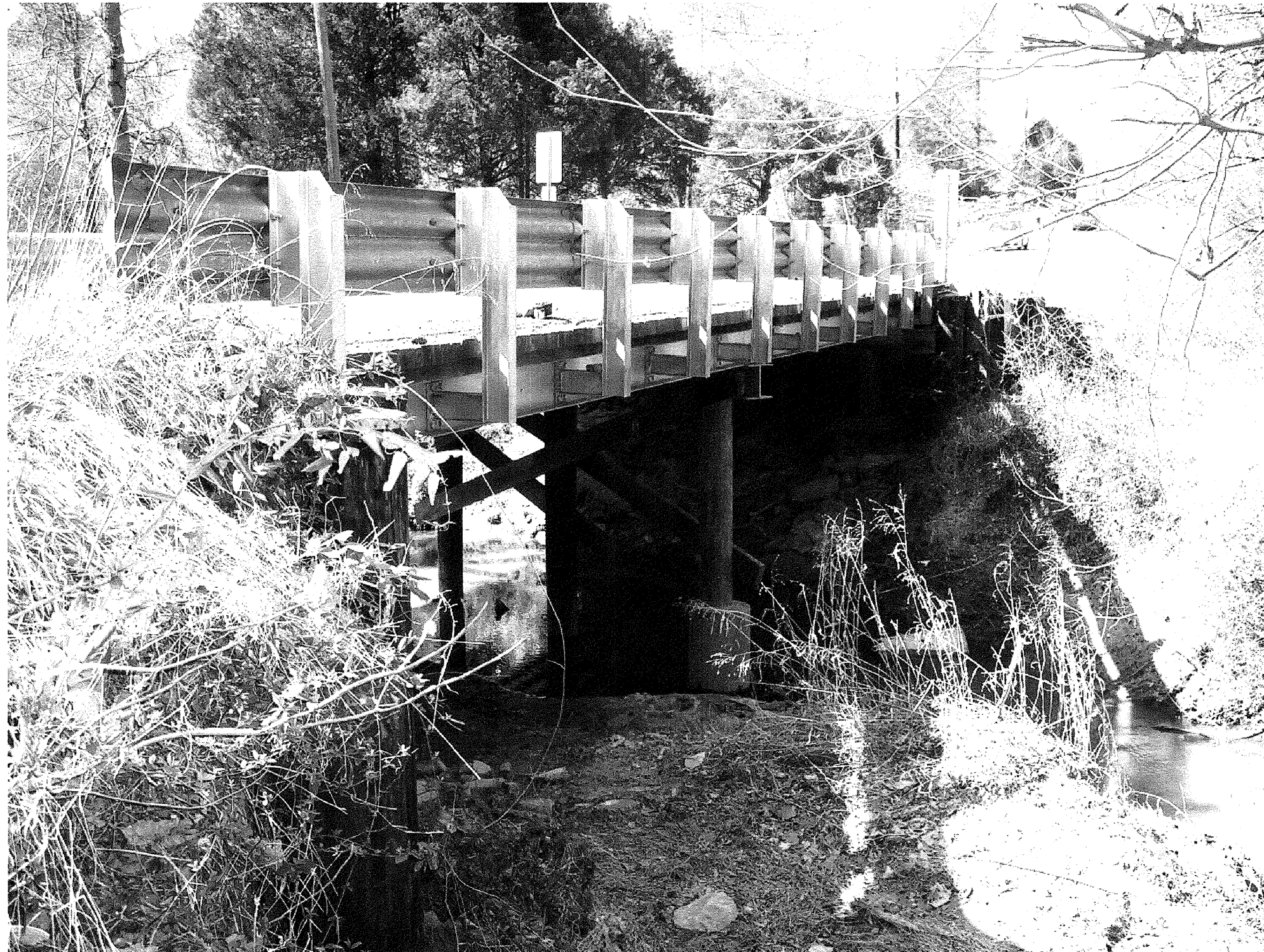
Looking East towards End Bent 1
