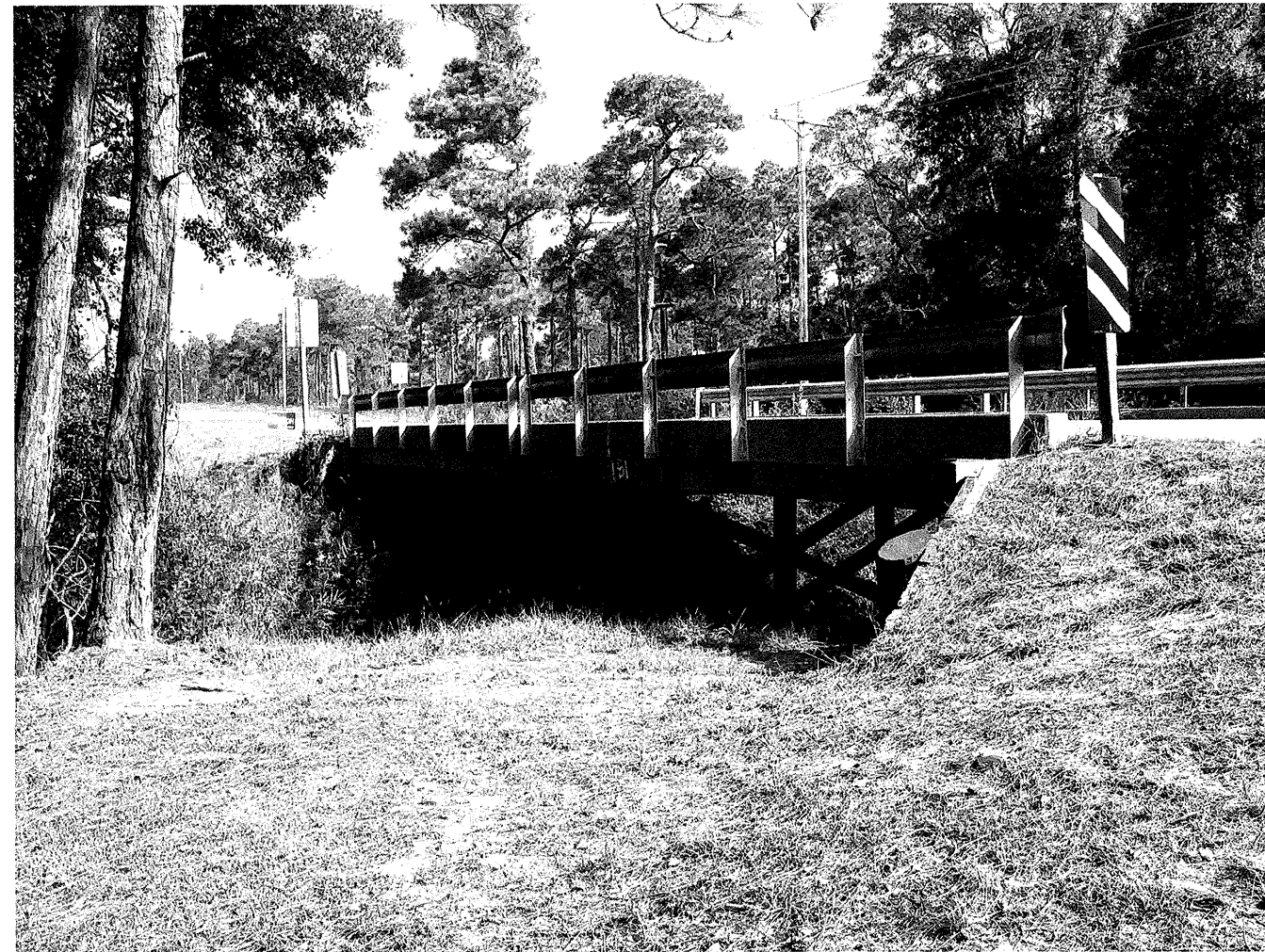
Looking north towards End Bent 2
