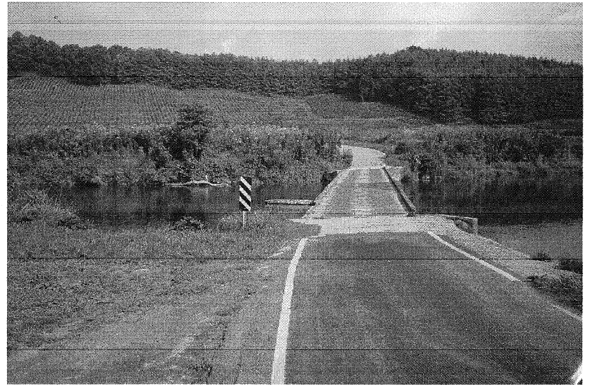
Looking Back From New End Bent 2
